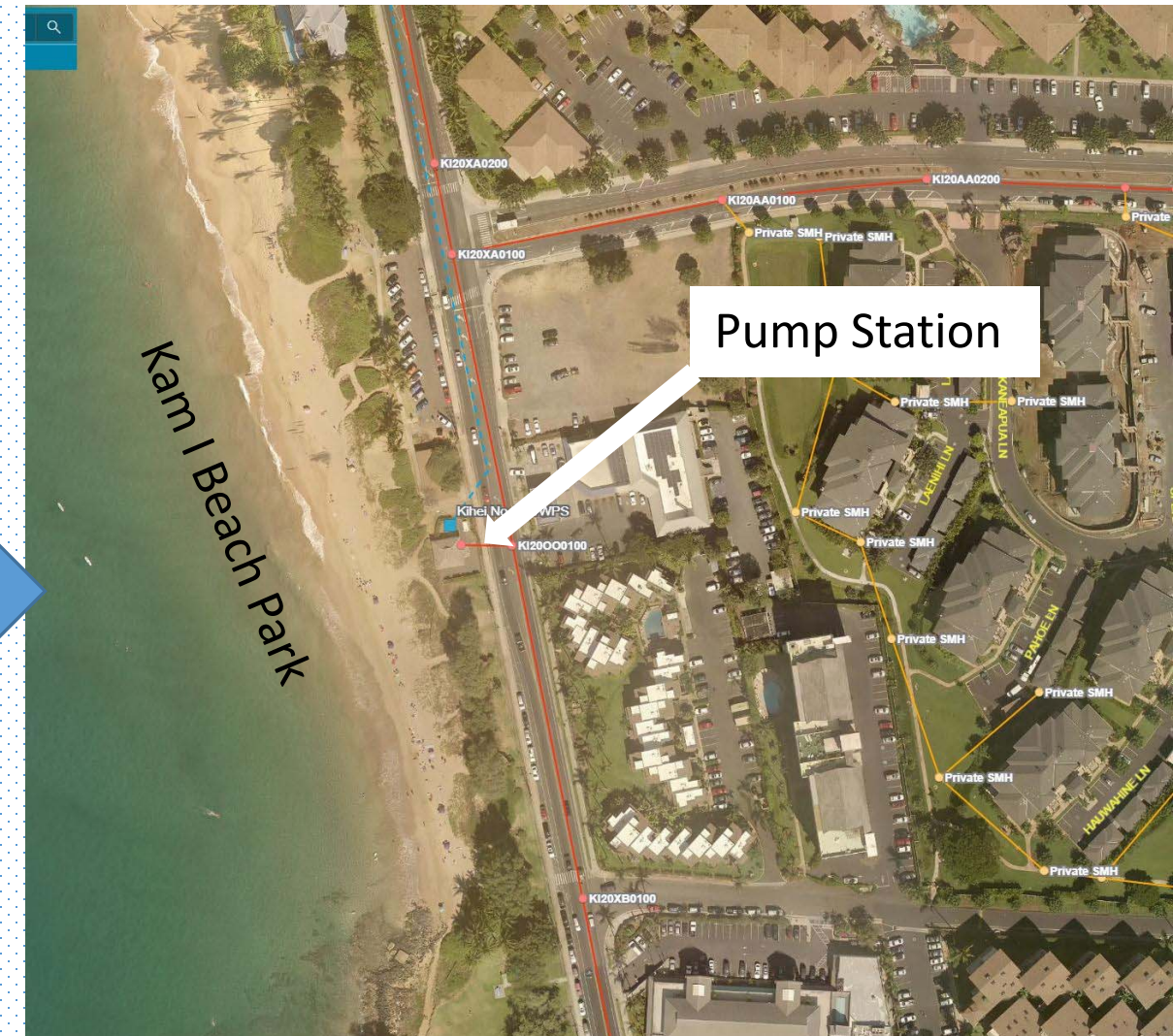
Kamaole I Beach Park and Kihei Wastewater Pump Station No. 7
