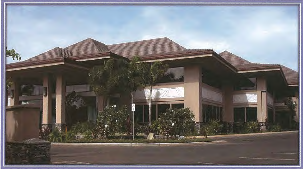
Commercial Condominium Units on Industrial Zoned Land – Commercial Classification
