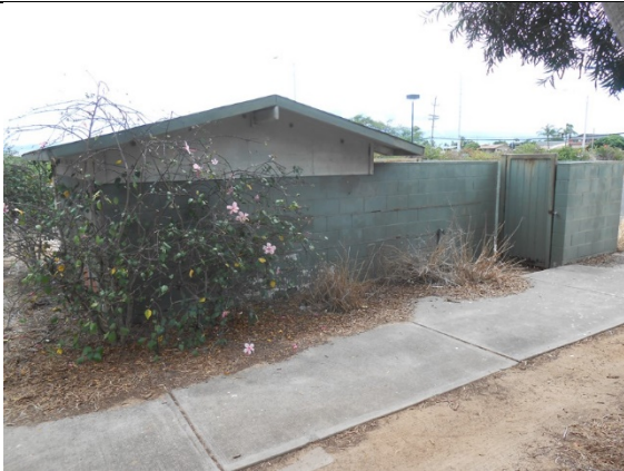
PTESB2: Overview of Trash Enclosure/Storage Building looking easterly.
