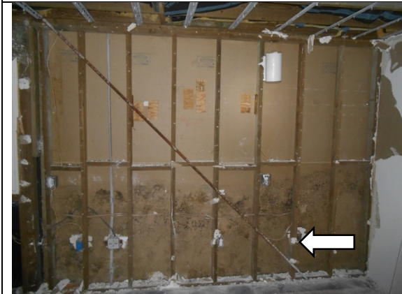
PA1CD.8: Discontinuous stud.
