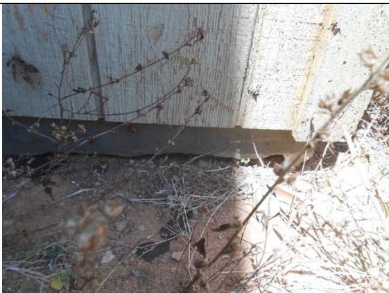
PB1CD.5: Exposed bottom of footing.
