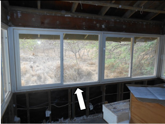
PC2CD.2: Wide opening with single sill plate.
