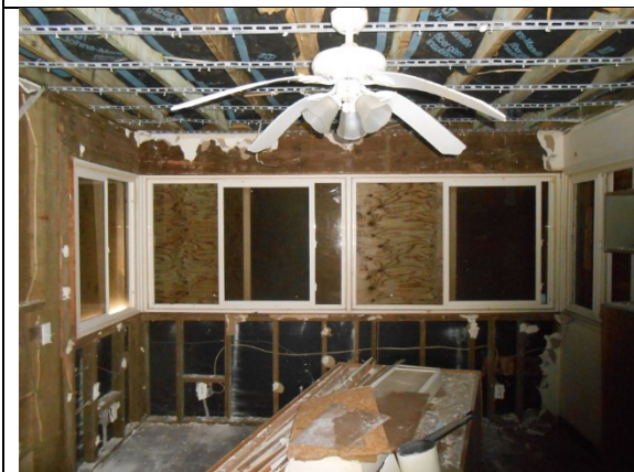
PB1CD.2: Wide opening with single sill plate.
