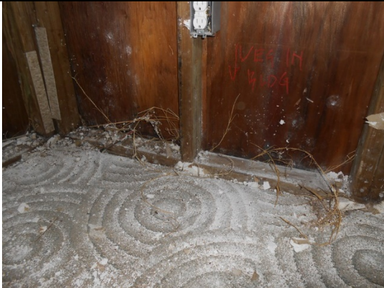
PA1CD.3: At various locations, vegetation is present at interior face of first story walls.
