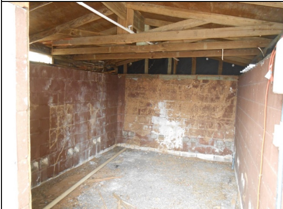
PTESB5: Interior view of storage building.
