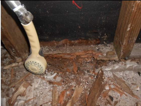
PA1D.4: Sole plate dry rot.
