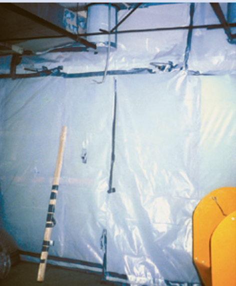
Photo 8: Full containment on large job
