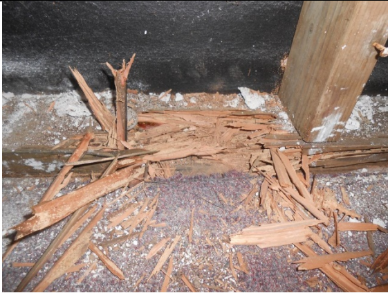
PB1D.1: Sole plate dry rot.
