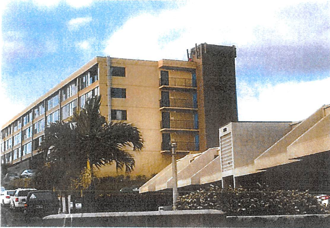
South Towards Site
