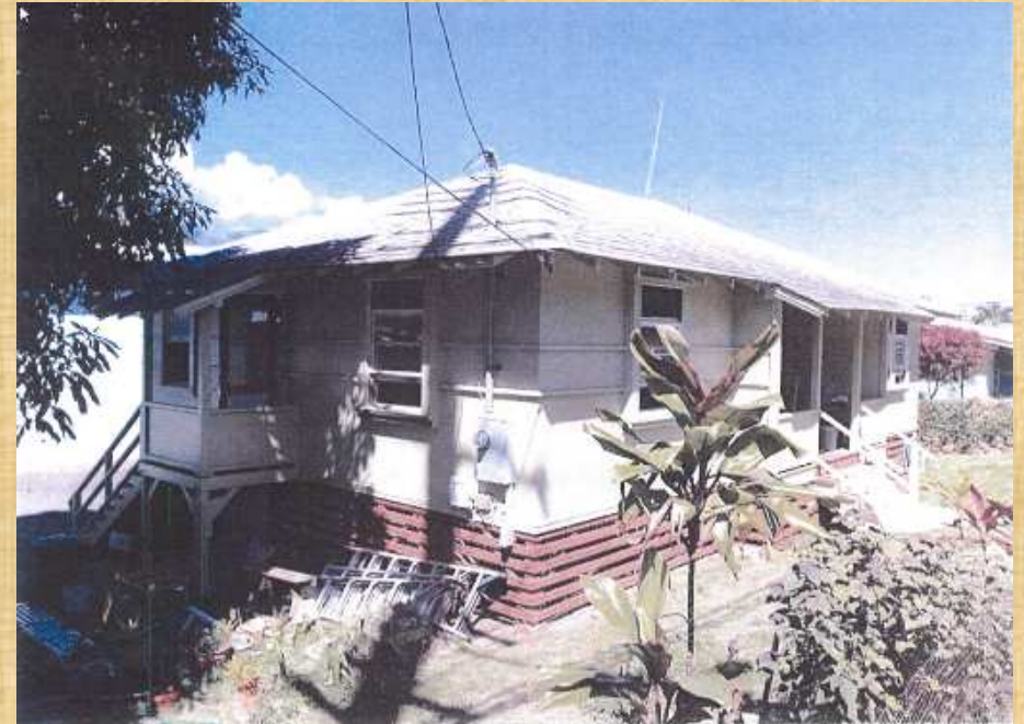
Front and Side View of the House
