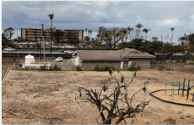
P.S. 3 – extensive wind and fire damage
