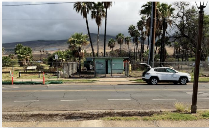
P.S. 5 – extensive wind and fire damage
