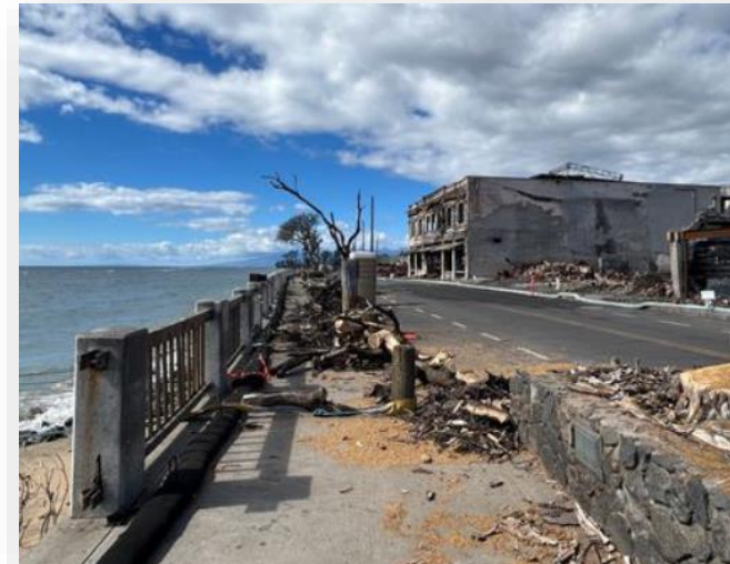
Front Street railing damaged
