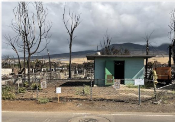
P.S. 6 – extensive wind and fire damage
