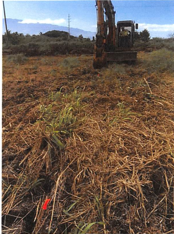
Figure 12. Overview Photograph of Proposed TR1 (View to Southwest)
