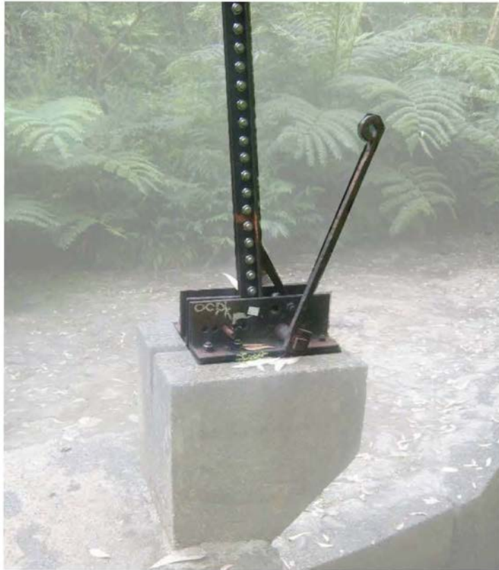
Figure 24: This typical ratchet type sluice gate operating mechanism is located at EMI Hoolawaili Stream diversion, on a tributary of Hoolawa, which is ordered to be restored as a "Habitat Stream" by CWRM. View facing SE. (Source: MAI, 2018.)
