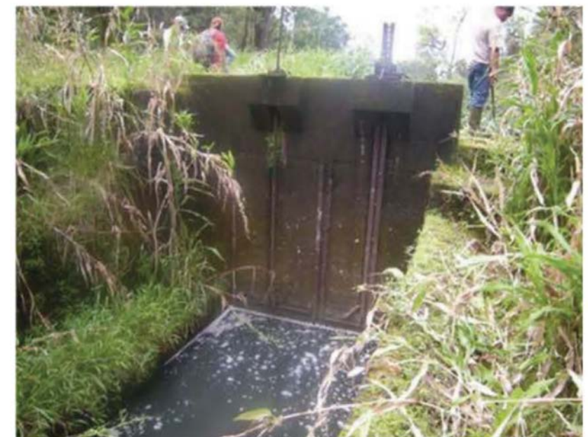
Figure 35: Another view of the threaded shaft gate mechanism at left. This gate is paired with a ratchet type gate. (Source: MAI, 2018.)
