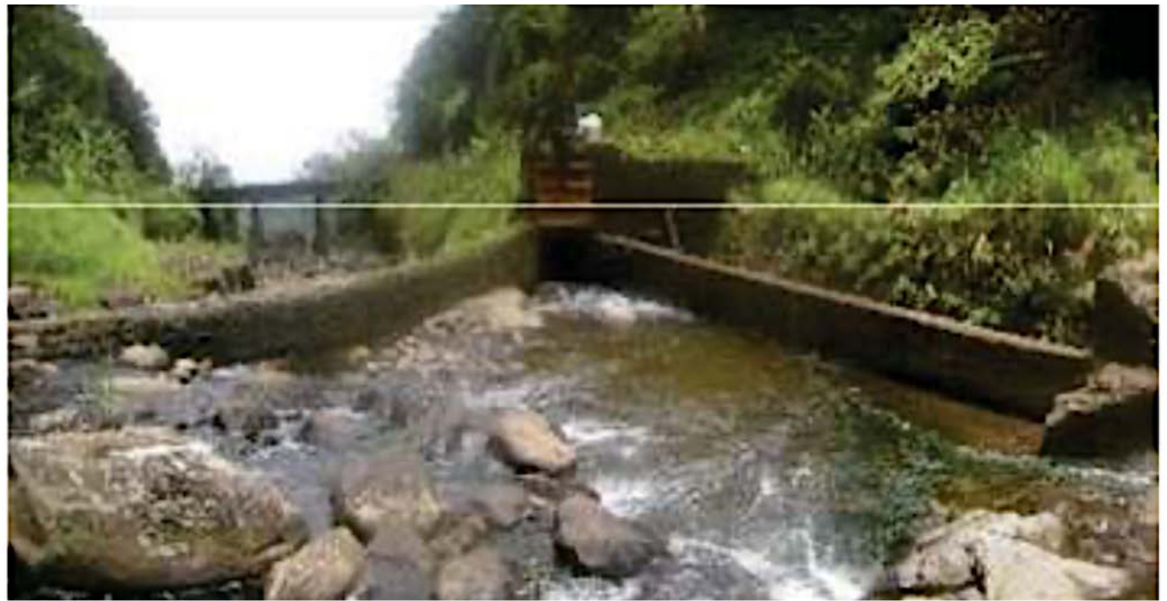
Figure 12: Honomanu Stream diversion. View facing E. (Source: MAI, 2018.)
