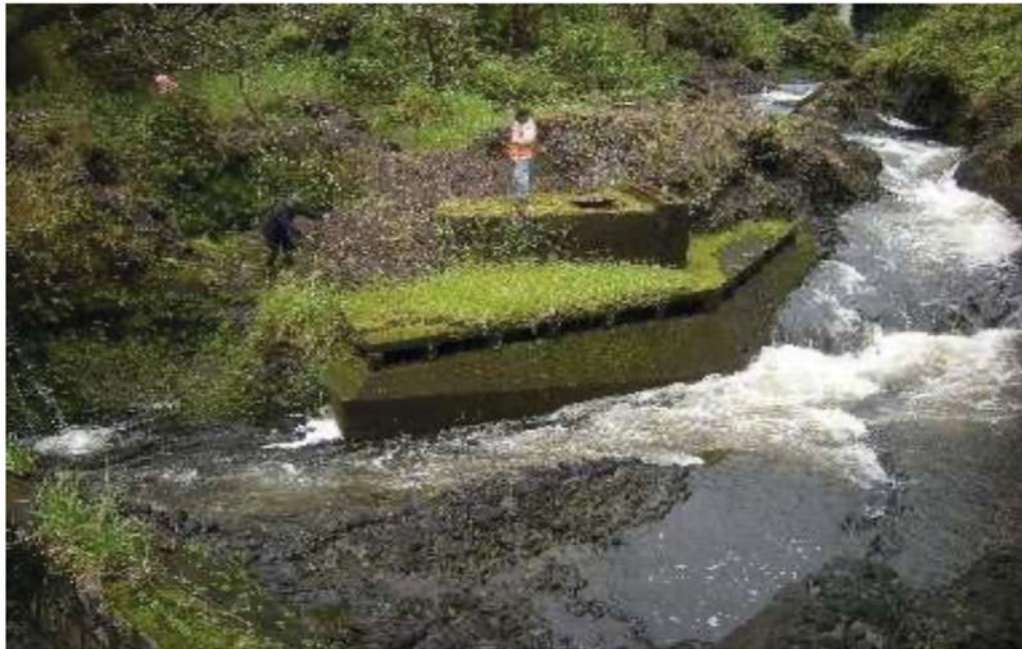
Figure 10: Intake at Hanawi Stream diversion. View Facing S. (Source: MAI, 2018)
