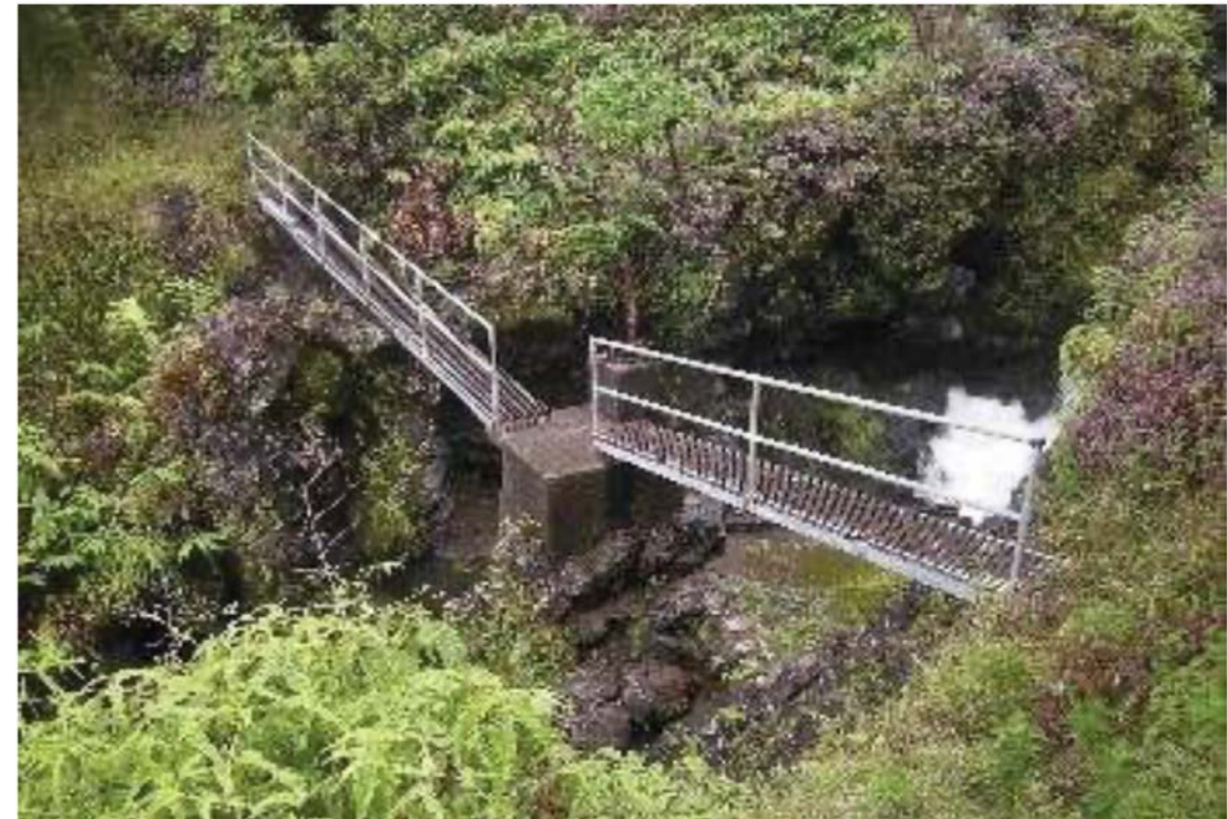
Figure 14: Walkway above Makapipi Stream diversion. View facing S. (Source : MAI, 2018.)
