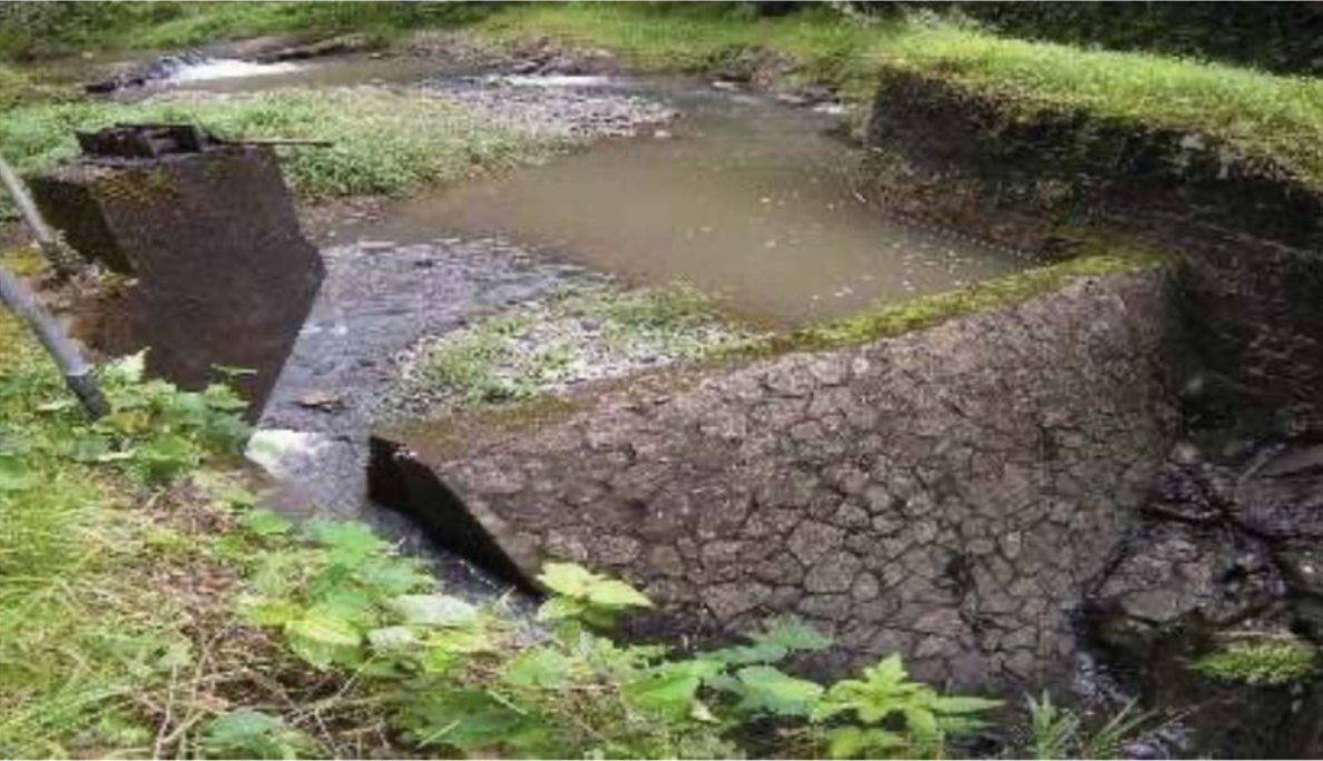
Figure 7: Dam at Wailuanui West Stream diversion impounds stream water for intake. (Source: MAI, 2018)
