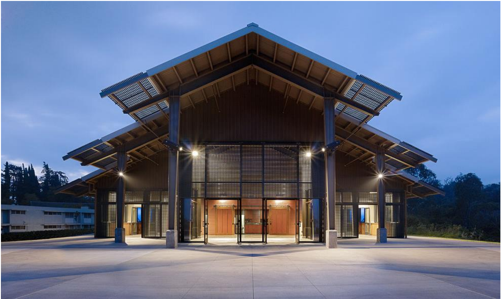
Photo 1: Creative Arts Center - view toward front entrance of main structure Image: Matthew Millman Photography
