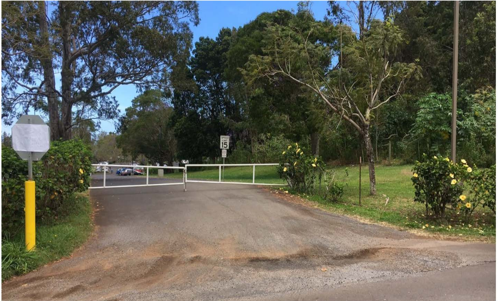
Hanamu Road Entrance - view of driveway towards parking lot (grassed and paved) on parcel 41
