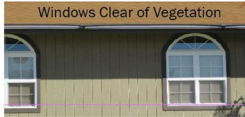
**Figure 35.** *Keep windows free of vegetation to reduce likelihood of heat-caused breakage that lets embers into your home.*
