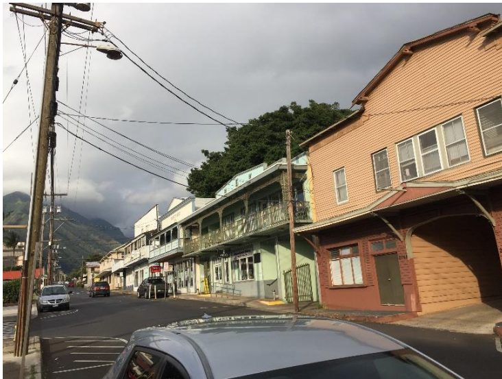
Vineyard Street adjacent to the PEF site
