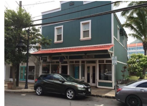
Existing retail on Market Street
