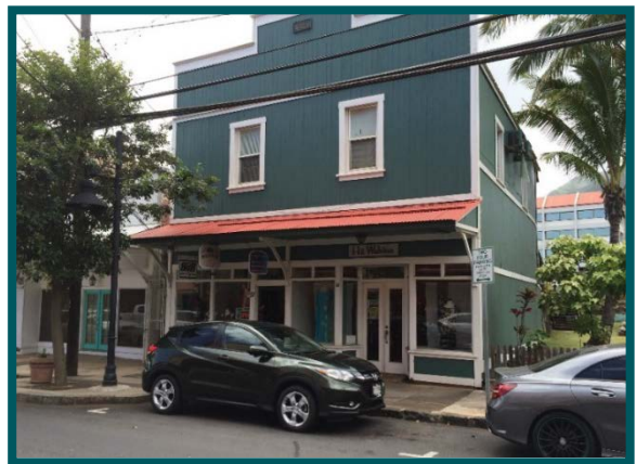
Existing retail on Market Street
