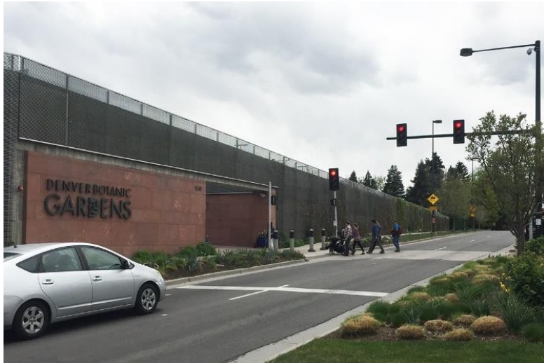
Denver Botanical Gardens, CO | Partial underground parking
