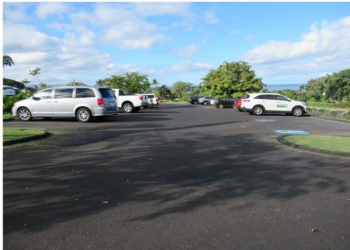
3. Looking west towards the ocean from within the Wailea Tennis Club Parking Lot. Two (2) ADA stalls with access aisle are seen on the right.
