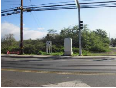
Welakahao intersection with main road, heavy fuels and power lines
