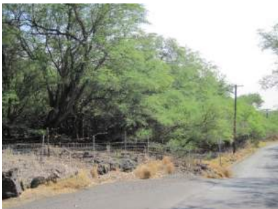
Vegetation overgrowing powerlines is a high hazard
