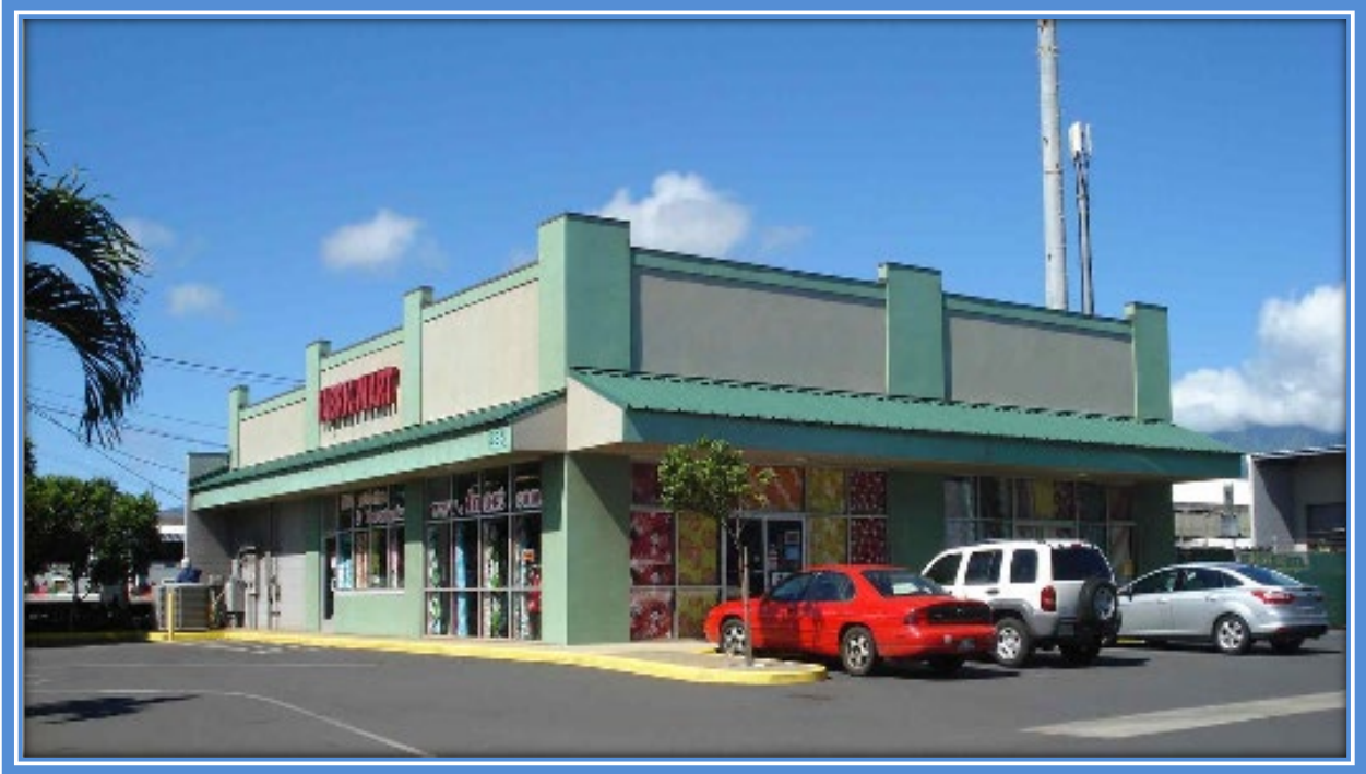
Commercial Store on Industrial Zoned Land – Industrial Classification
