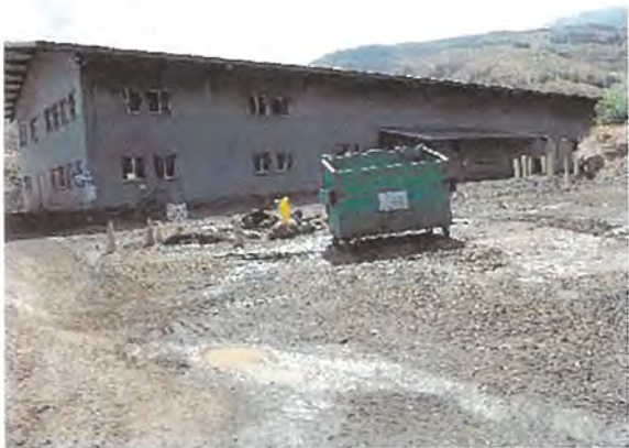
Gravel Roads with Mud and Erosion
