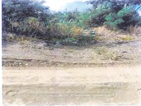
Road Crossing Pohakea Lacking BMPs
