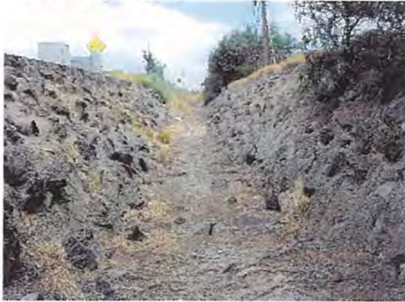
Waihe'e Makai Ditch – Armored and Box Cut
