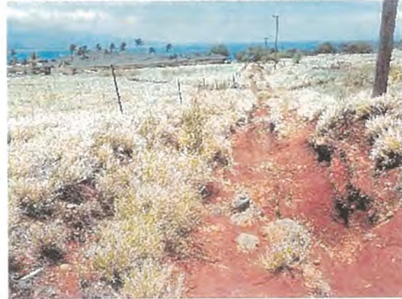
Distribution Lines and Failed Roads
