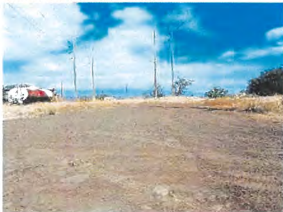
Well Maintained Gravel Roads
