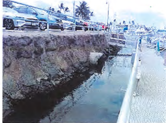
Culverts Discharging into Harbor
