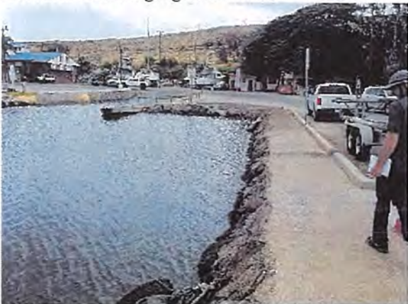
Culvert Outfall to Harbor
