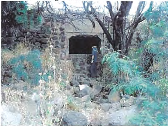
Culverts Discharging into Harbor
