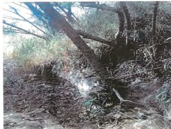
Wrack Lines and Eroded Bank within Pohakea
