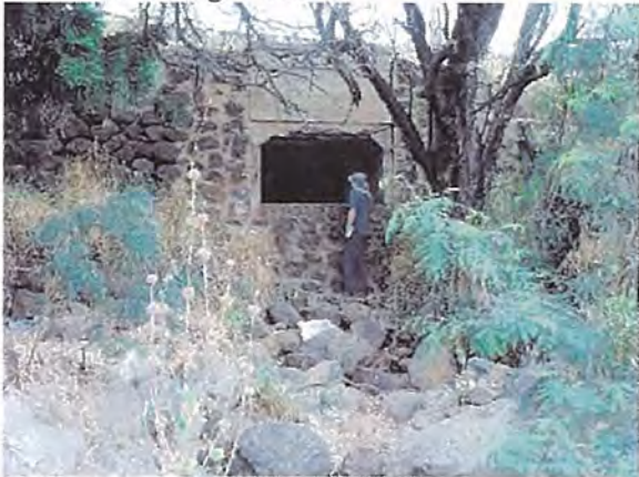
Culverts Discharging into Harbor
