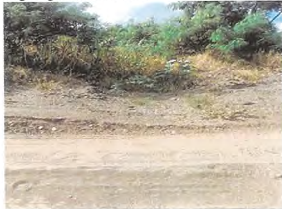
Road Crossing Pohakea Lacking BMPs
