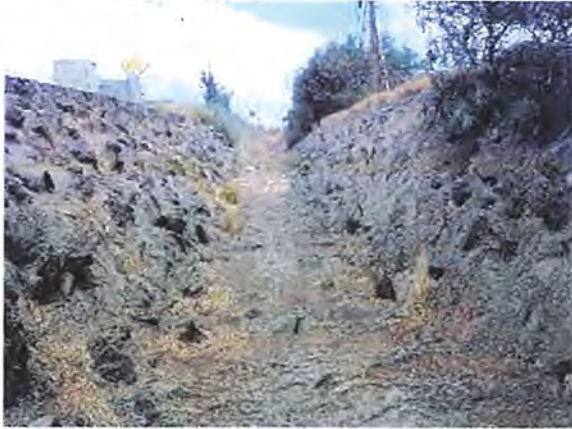
Waihe'e Makai Ditch – Armored and Box Cut
