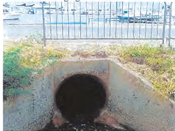
Culverts Discharging into Harbor
