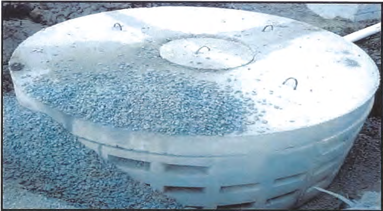
Figure 28. Stormwater Infiltration Well
