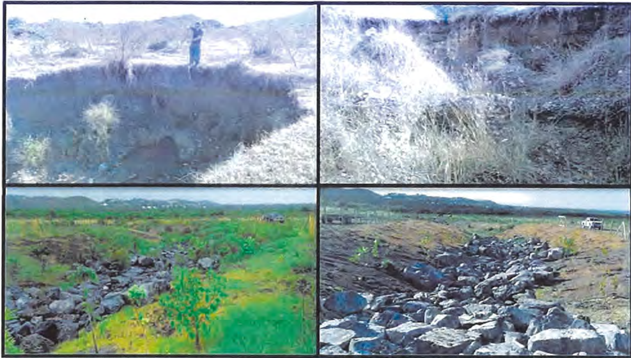
Figure 22. Examples of Head Cutting and Stabilization
