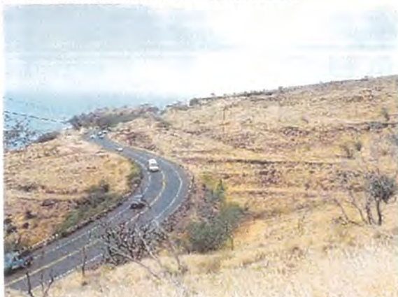
Transmission Lines along the Pali
