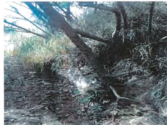
Wrack Lines and Eroded Bank within Pohakea
