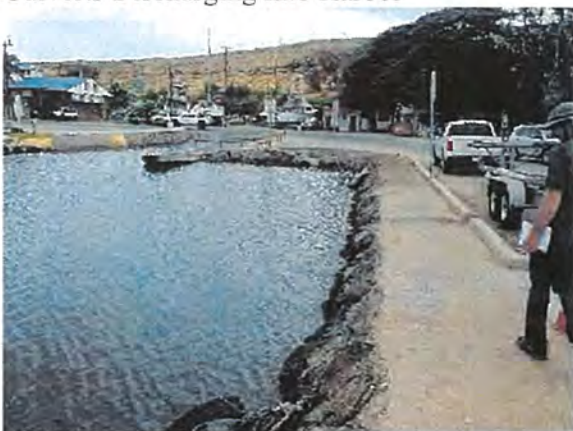
Culvert Outfall to Harbor
