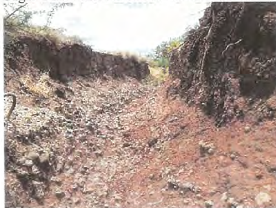
Highly Eroded Stream Channel
