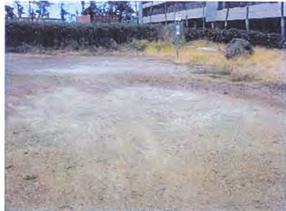
Dirt Lots with No BMPs in Place
