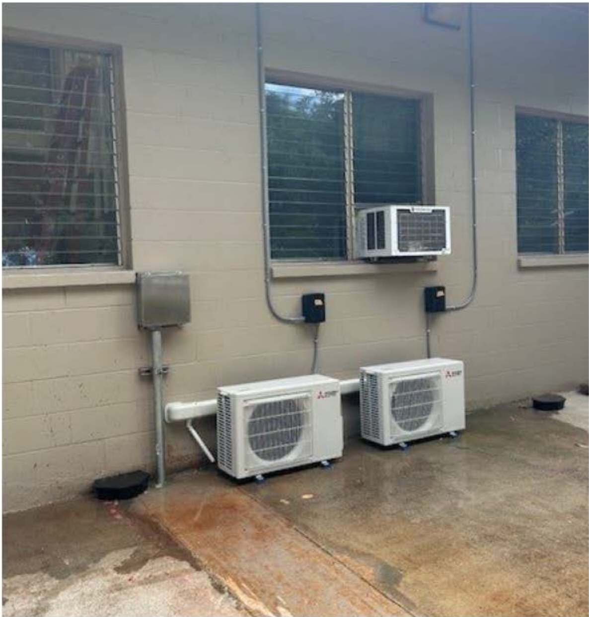
LANAI FIRE STATION HVAC INSTALLATION
