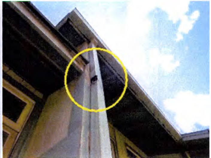
Damaged/broken/missing gutters noted. Recommend having a licensed contractor evaluate and repair/replace as necessary.
