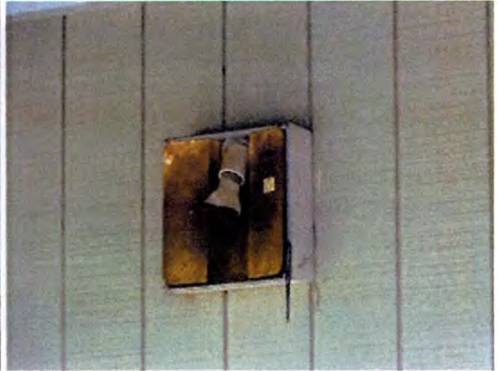
Some of the exterior lighting fixtures were damaged and need to be replaced.
