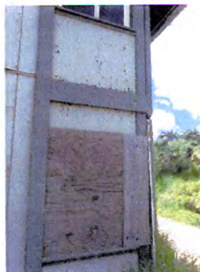
Many of the ground floor windows were broken at the time of inspection.
