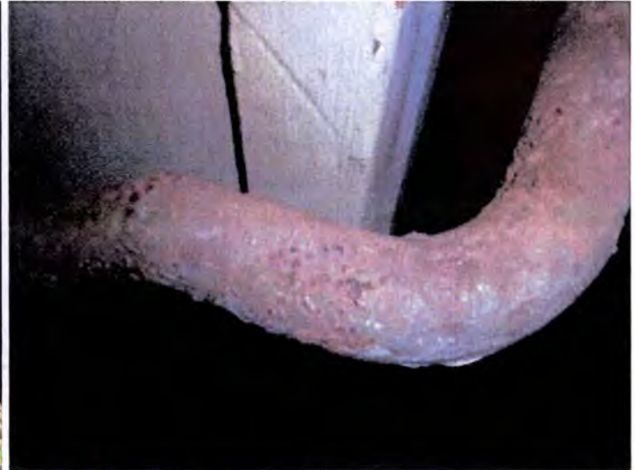
Exterior stair handrails were corroded and need to be cleaned, treated and refinished.
