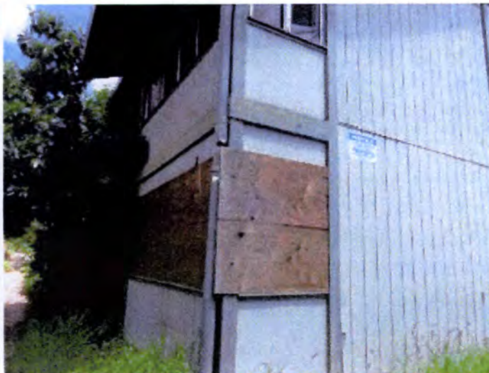
Many of the ground floor windows were broken at the time of inspection.
