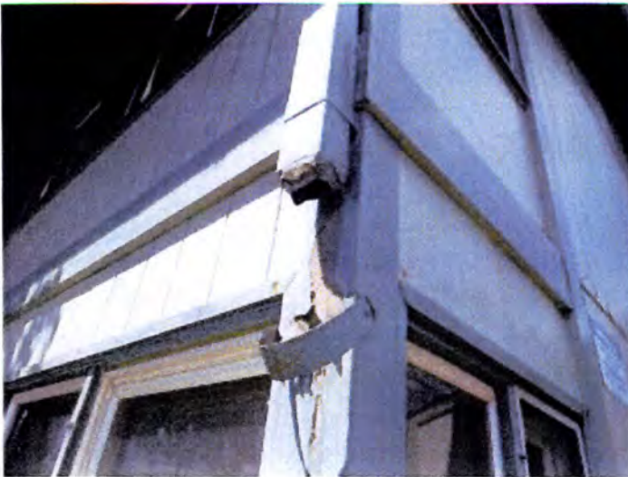
Damaged/broken/missing gutters noted. Recommend having a licensed contractor evaluate and repair/replace as necessary.
