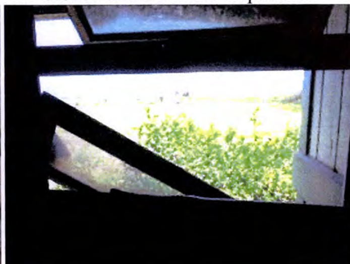
The stair way windows were heavily corroded, damaged and/or inoperable at the time of inspection. Recommend replacement.
