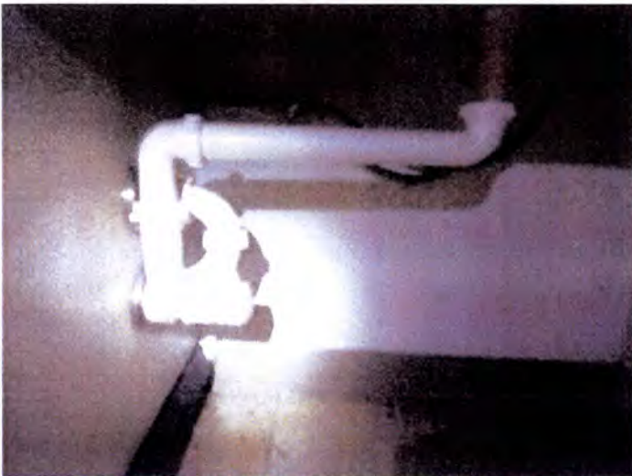
ABS/PVC waste/drain plumbing
