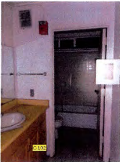
3.7: Interior Elements 3.7.6: Bathrooms
