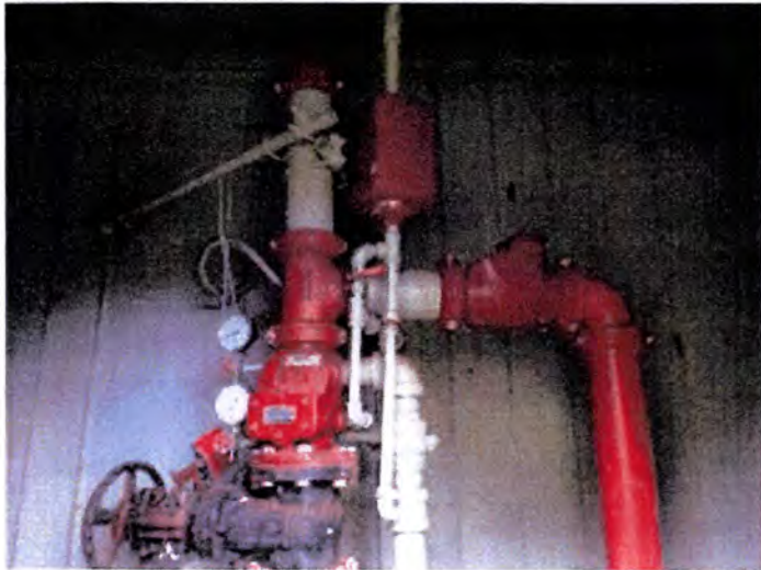
Sprinkler Systems: due to the system not having been properly serviced at required intervals, adequacy or performance questionable.
