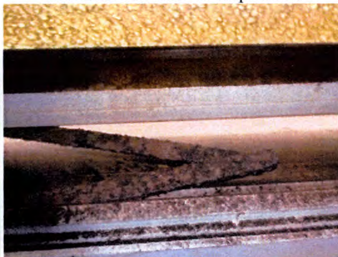
The stair way windows were heavily corroded, damaged and/or inoperable at the time of inspection. Recommend replacement.
