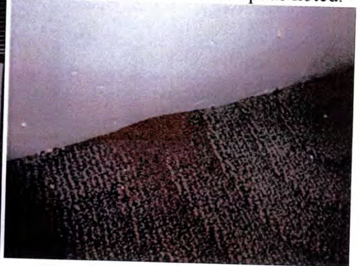
There were visible indications of moisture and termite damage observed at the interior window trim areas. Recommend replacement of all interior window trim and finishes.
