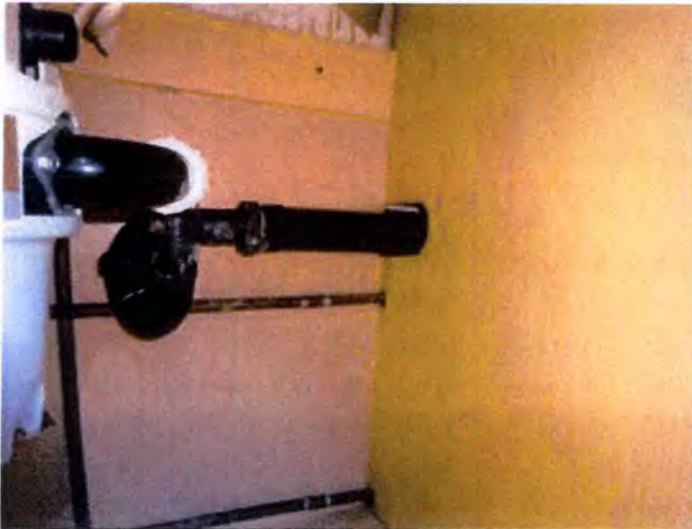
ABS/PVC waste/drain plumbing
