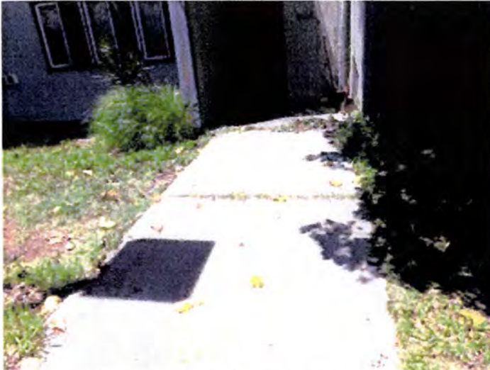
Concrete sidewalks noted.
