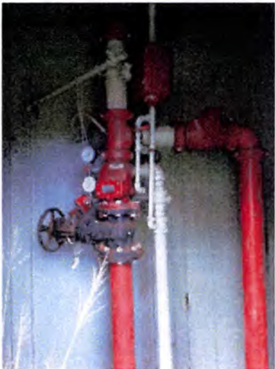
The installed risers and associated equipment appeared to be damaged/improperly maintained when inspected. Recommend having a licensed fire suppression contractor evaluate, service, test and inspect the entire fire suppression system.
