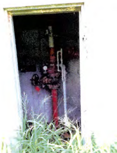
The fire suppression risers were located at the end of each building.
