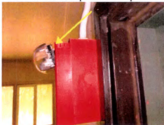
Approximately half of the installed pull stations were damaged when inspected. Recommend replacement/repair.
