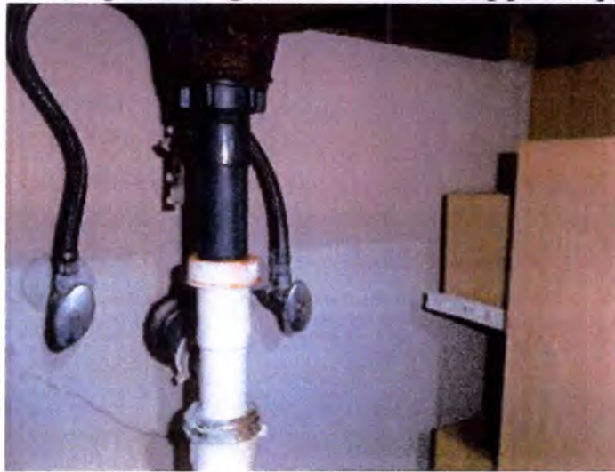
ABS/PVC waste/drain plumbing
