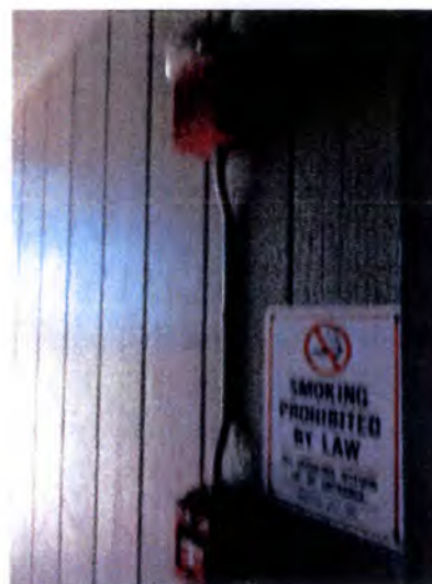
Approximately half of the installed pull stations were damaged when inspected. Recommend replacement/repair.
