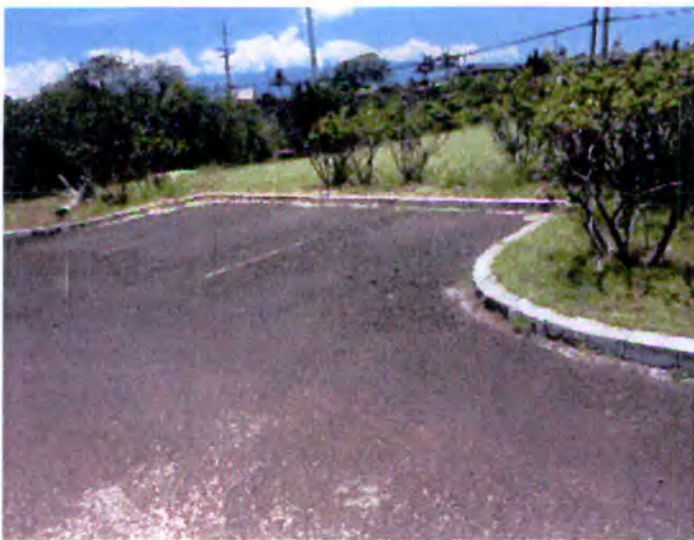
The parking area surface was deteriorated with lines weathered to the point of not providing clear lanes for parking use. Recommend having the parking area resurfaced and striped to ensure proper identification of parking stalls.
