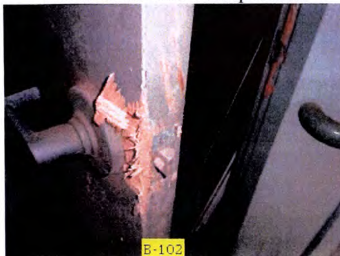
The exterior doors were termite damaged or deteriorated to the point of being inoperable. We recommend replacement of all exterior doors, framing and trim for all buildings.
