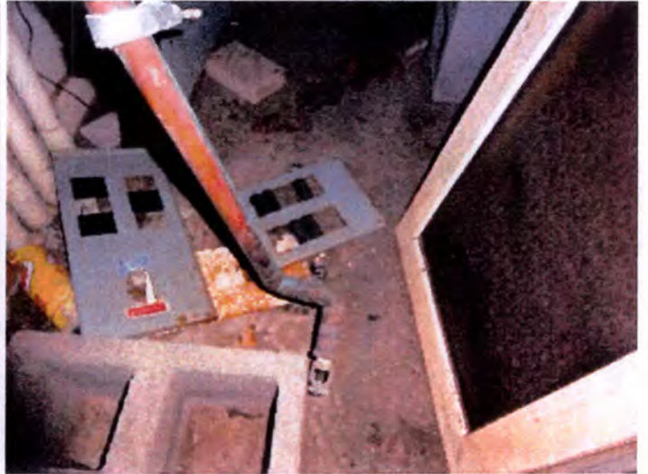
Building B: Sprinkler branch pipe was broken/bent down in the electrical room. Recommend repair.
