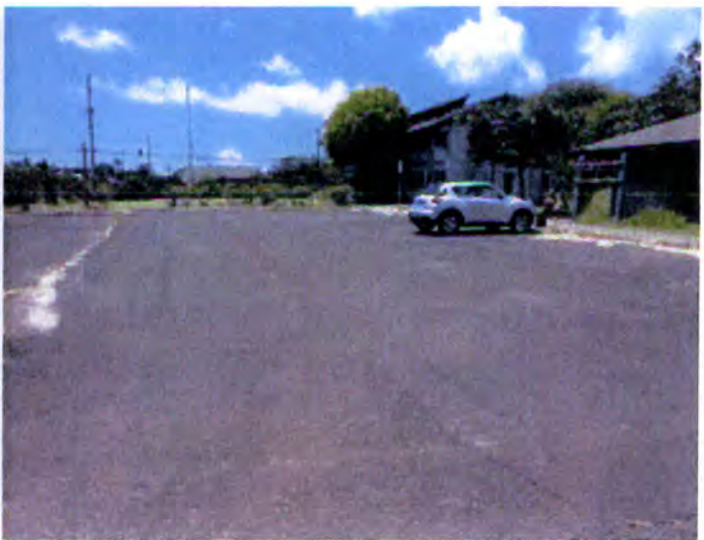
The parking area surface was deteriorated with lines weathered to the point of not providing clear lanes for parking use. Recommend having the parking area resurfaced and striped to ensure proper identification of parking stalls.
