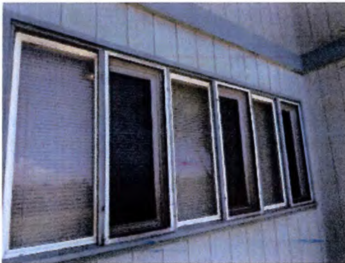
Vinyl framed windows noted
