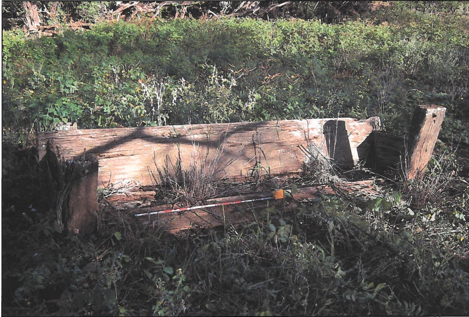
Figure 32: View North of State Site 50-50-14-7900 Showing Wood Trough.
