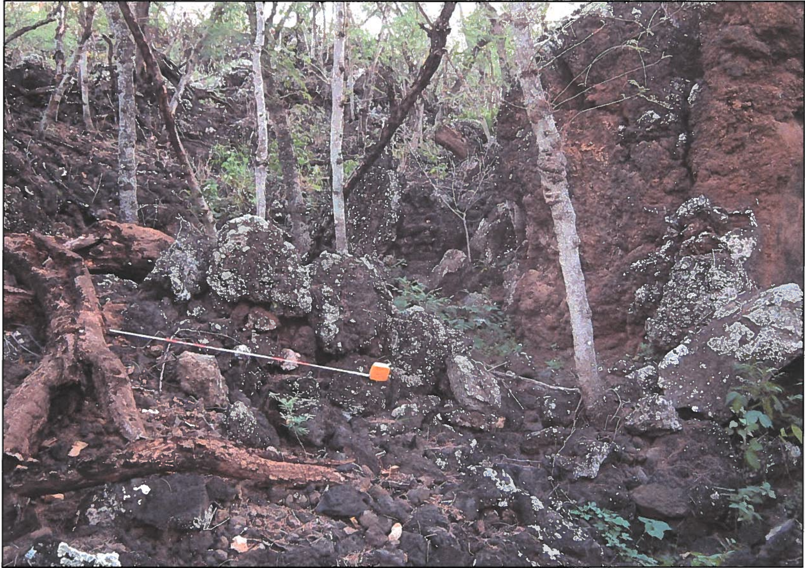
Figure 53: View Southwest of State Site 50-50-14-7915 Showing Water Diversion Wall.
