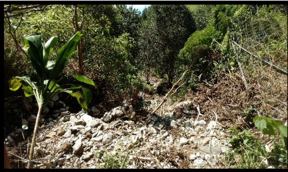
Photos above: An example of the effects of the September storm: A five meter section of the SE7a fence in Hanaula was destroyed by high water (left). New posts were pounded and hog panels were installed to prevent future ungulate ingress (right).
