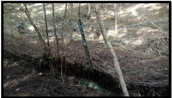
Photos above: The accumulation of debris on the SE5 fence in Hanaula following the September storm (left), and after maintenance (right) to alleviate the pressure of debris on the fence.
