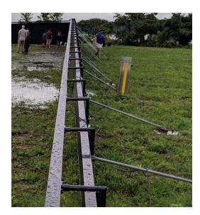
At the center point or apex of The Wall, the panels are slightly more than 7 ½ feet in height. Like The Wall, the panels slope from their apex height to 3-inches at the ends. The framework for these panels set on baseplates that are hammered into the ground using stakes approximately 18-inches in length.
