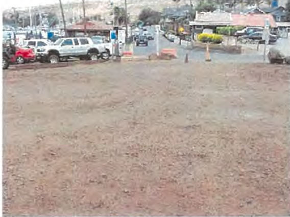
Dirt Lots with No BMPs in Place
