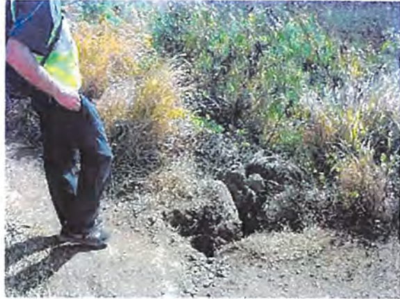
Erosion and Discharge from Road
