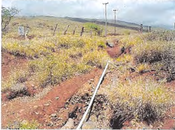
Channelization and Erosion
