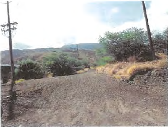
Gravel Roads Near Ditches
