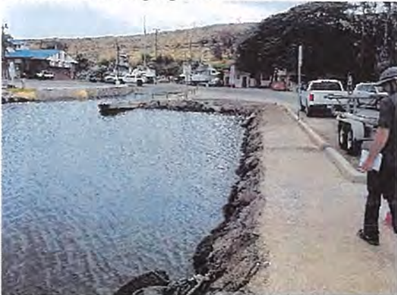
Culvert Outfall to Harbor
