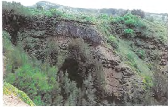
Loss of Vegetation
