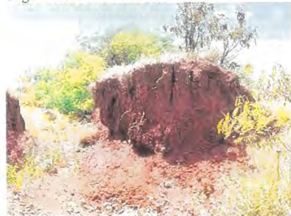
Evidence of Severe Erosion
