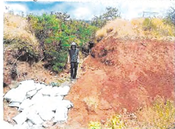
Sand Bags at Channel Outfall to Detention Basin
