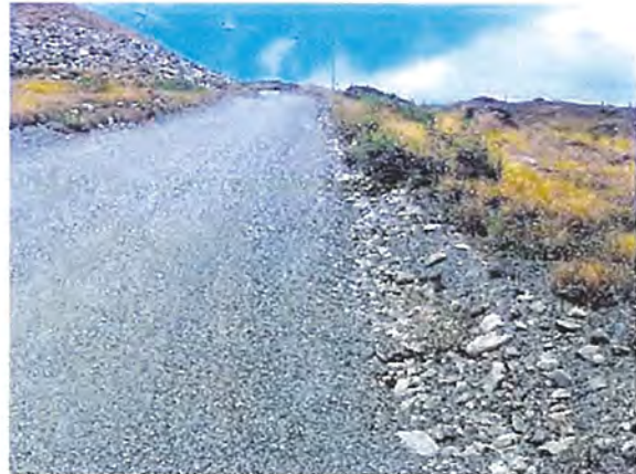
Well Maintained Road with Swale
