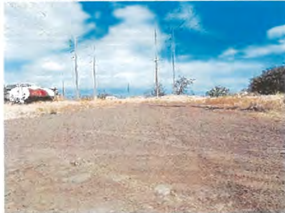
Well Maintained Gravel Roads
