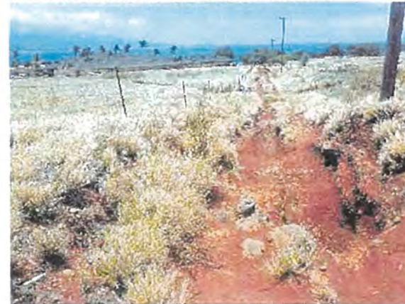
Distribution Lines and Failed Roads
