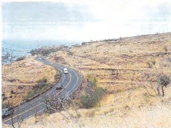
Transmission Lines along the Pali
