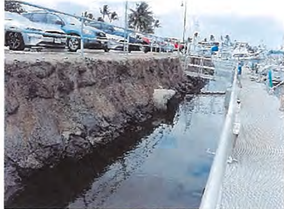
Culverts Discharging into Harbor
