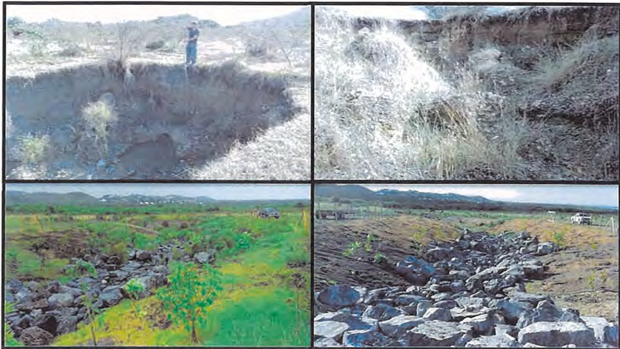
Figure 22. Examples of Head Cutting and Stabilization
