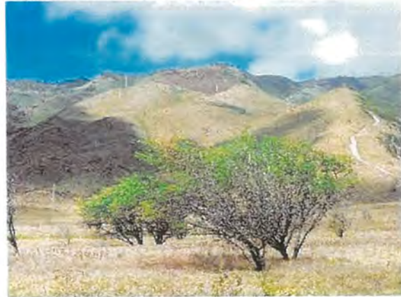
Transmission Corridor and Evidence of Fire
