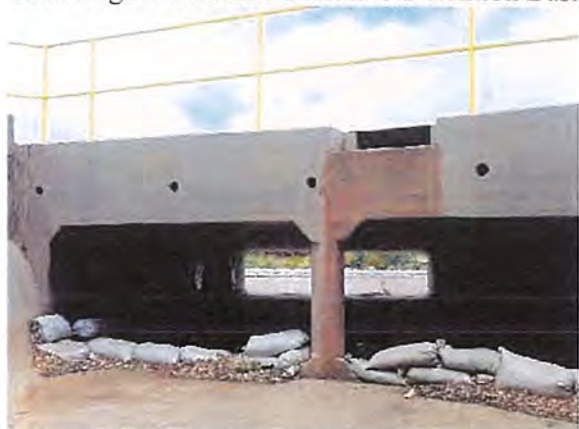
Sand Bags Under Hau'oli Street
