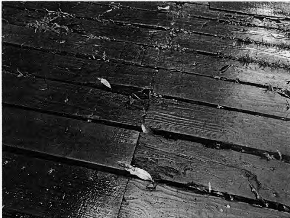
PHOTO 8 CLOSE-UP VIEW OF 4x12 TIMBER DECK PLANKS
