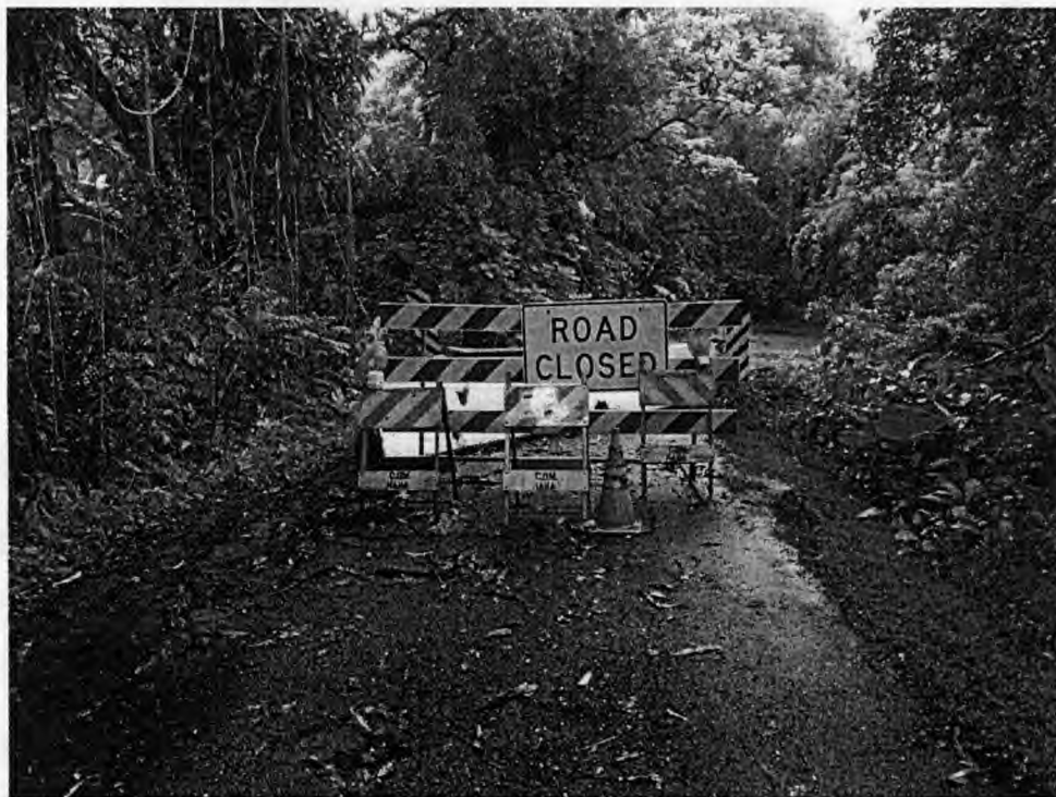
PHOTO 14 BARRICADE AT MAUKA END OF BRIDGE LOOKING MAKAI
