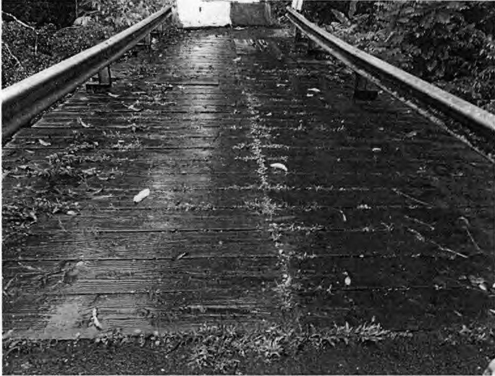
PHOTO 1 4x12 DECK PLANKS AND METAL GUARDRAILS ON BRIDGE
