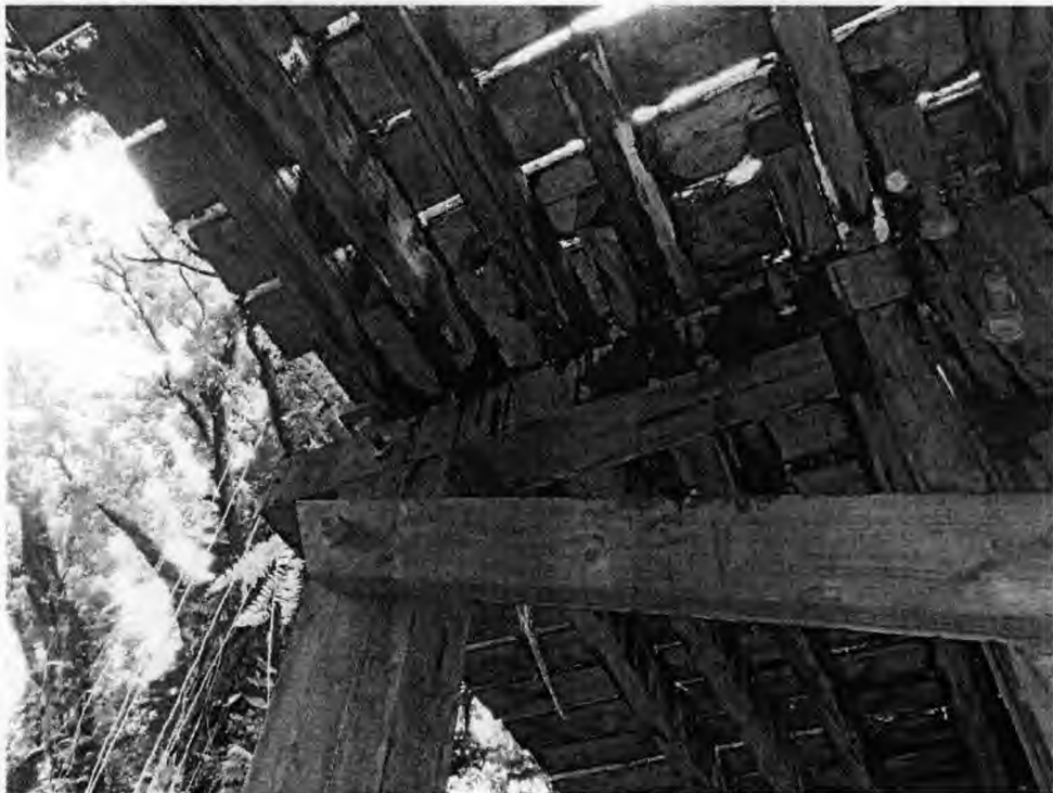
PHOTO 4 6x12 TIMBER GIRDERS LAPPED OVER INTERMEDIATE PIER
