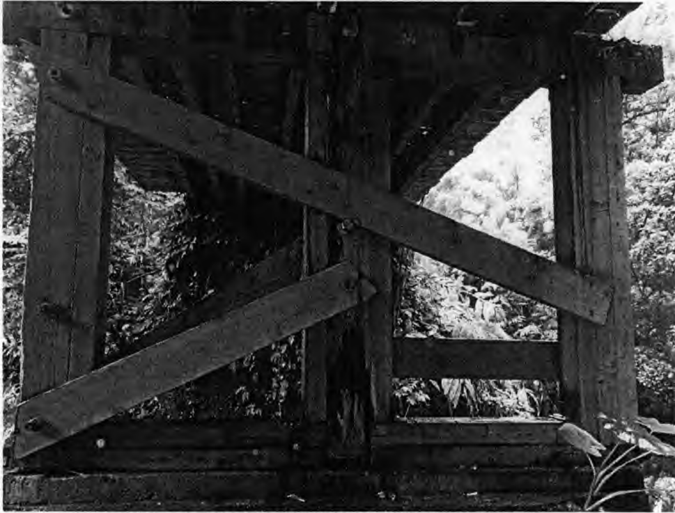
PHOTO 5 TIMBER PIER BETWEEN THE MAUKA AND MAKAI SPANS
