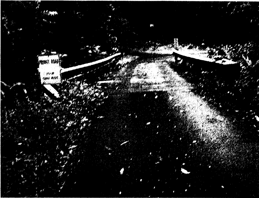
PHOTO 1 Mauka Approach to Bridge
