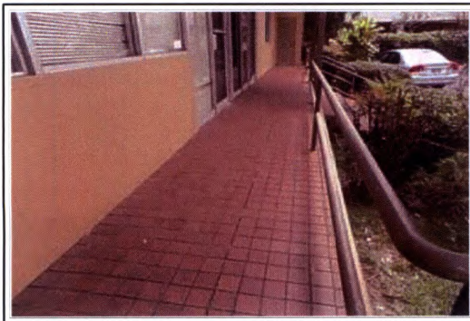
EVIDENCE OF SPALLING ON PORCH
