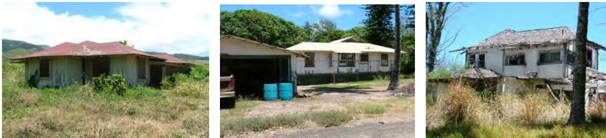
The three structures on the Waihe'e Coastal Dunes and Wetlands Refuge. Left: the C.W. Dickey home to be remodeled as MCLT's new cultural education center. Center: the old Waihe'e Dairy caretaker's house slated for renovation. Right: structure known as the doctor's house, which is slated to be demolished.
