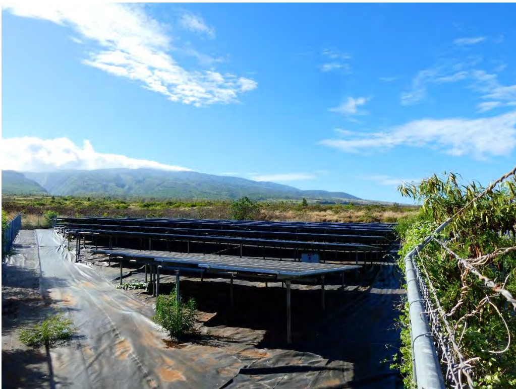
PHOTO NO. 4: Southeasterly view of the solar farm improvements.
