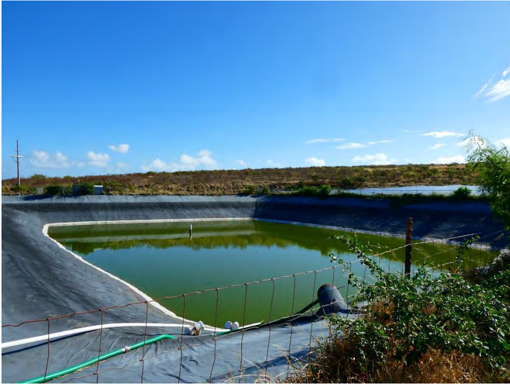
PHOTO NO. 3: Northeasterly view of the reservoir improvements.
