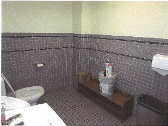
2nd Floor Interior
