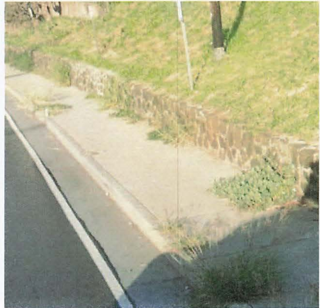
Vegetation growth in cracks of newly constructed sidewalk at Mill Stret and N. Market Street. Google Earth. February 2025.
