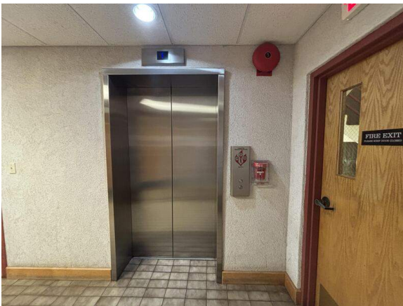
45 Typical elevator doors
