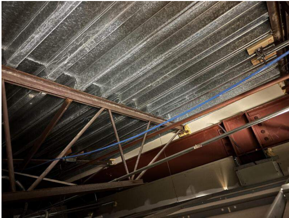
19 Underside of typical upper level
