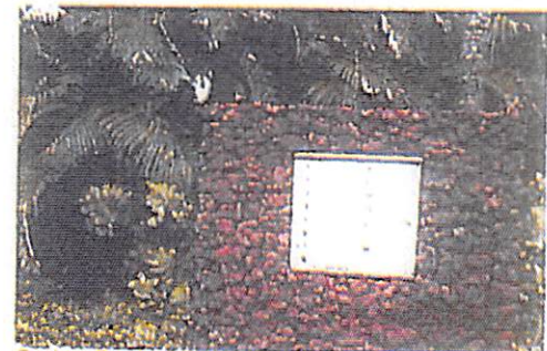
Custom Box installed by Developer
