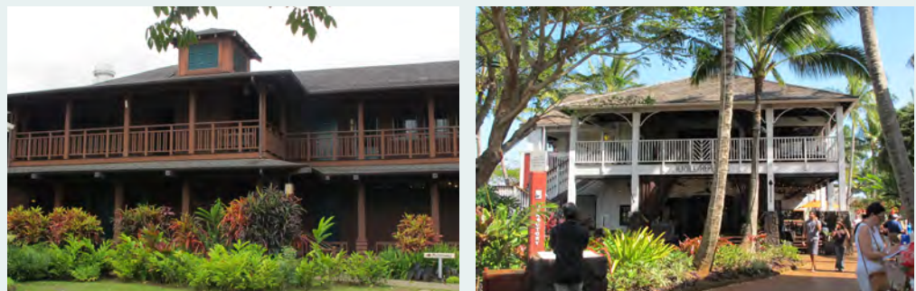
Figure 5.1 Examples of Maui's vernacular architectural style that incorporates design elements to address local climate.
