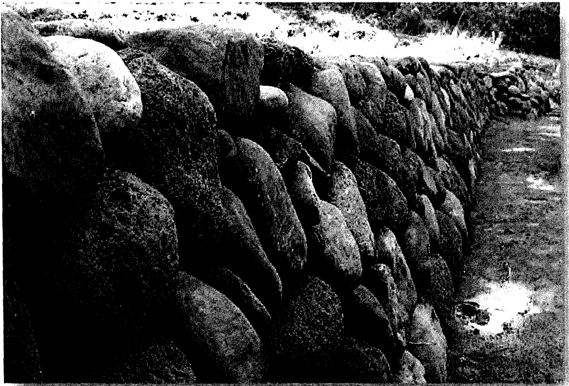
Figure 42: Lo'i Kalo Wall Restoration at Noho'aha Farm, Waikapū - Hōkūao Pellegrino (2005)
