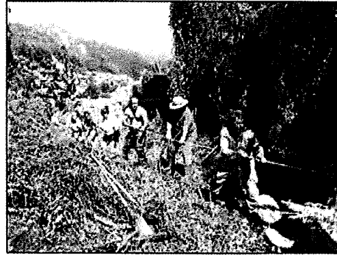
Figure 15: Waikapū ‘Auwai Restoration - Hōkūao Pellegrino (2004)
