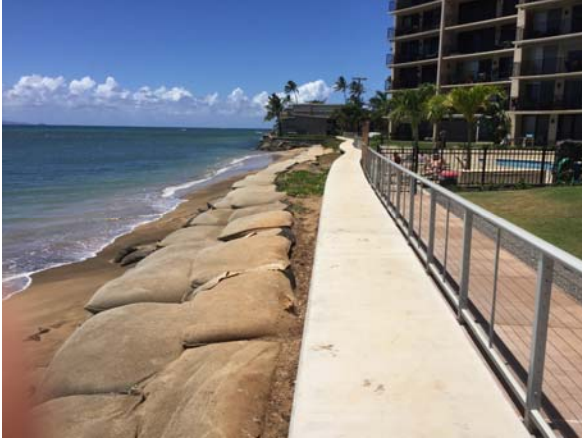
Hololani, 2019. Sheet pile seawall with concrete cap is installed.
