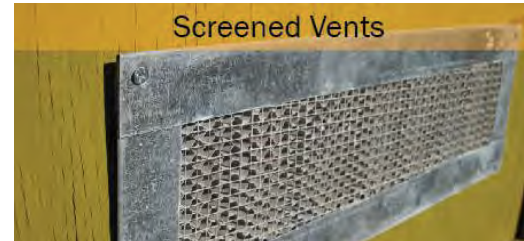
Figure 6. Covering vents with 1/8-inch or smaller metal mesh blocks embers from entering a home or structure.
