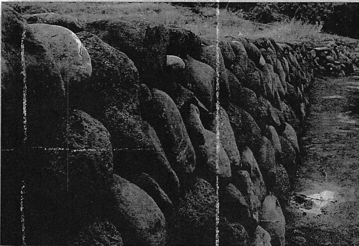
Figure 42: Lo'i Kala Wall Restoration at Noho'ana Farm, Waikapū - Hokūao Pellegrino (2005)
