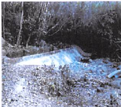
Figure 28. Waikapū Dam Intake Diversion (2012)
