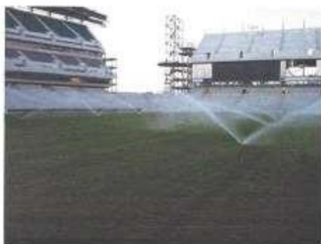
2. Underground, automatic irrigation system (photo: T.J. Semashk)
