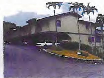
Photo 13: Building E, 16 units.
