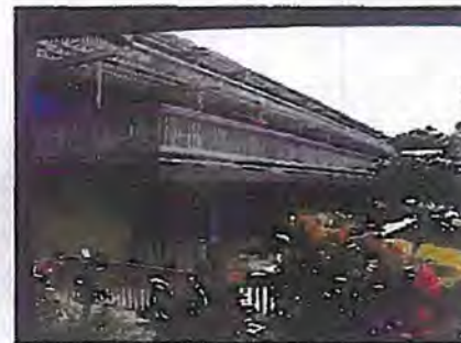
Photo 10: Building B, 16 units.
