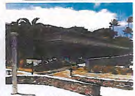
Photo 14: Building F, 12 units.
