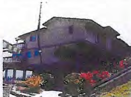
Photo 9: Building A, 10 units.
