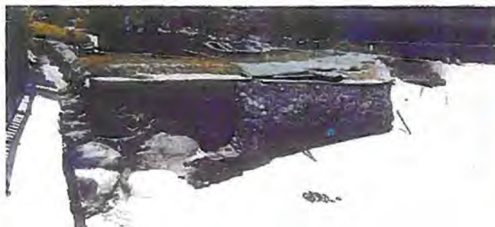
Photo 28: Existing seawall at 36-inch drainage outfall. Outfall will be relocated approximately 3-feet inland. Green plywood covers sink holes behind seawall.
