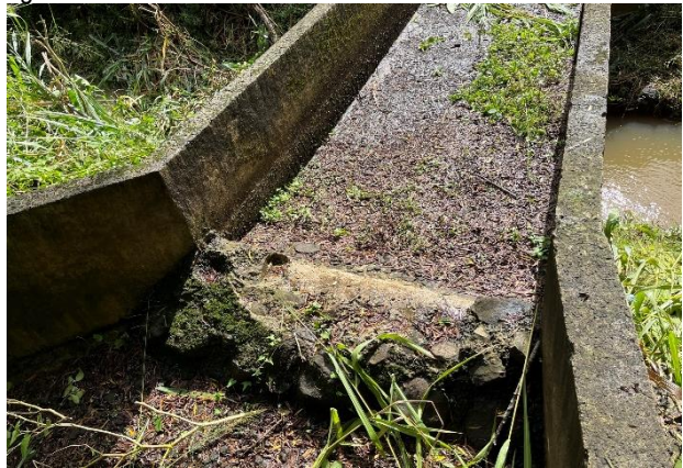
B) East Kuiaha Stream bypass over Kauhikoa Ditch.
