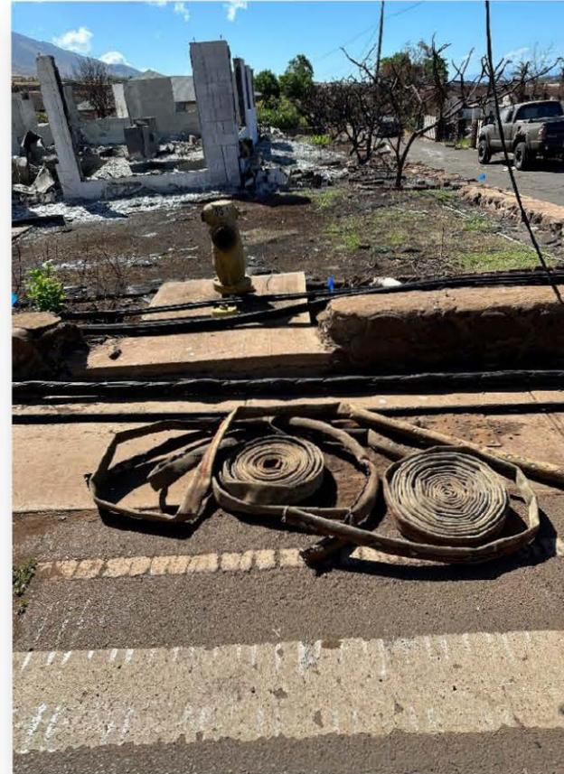
*Fire hydrants, water meters, and water laterals will need to be replaced*
