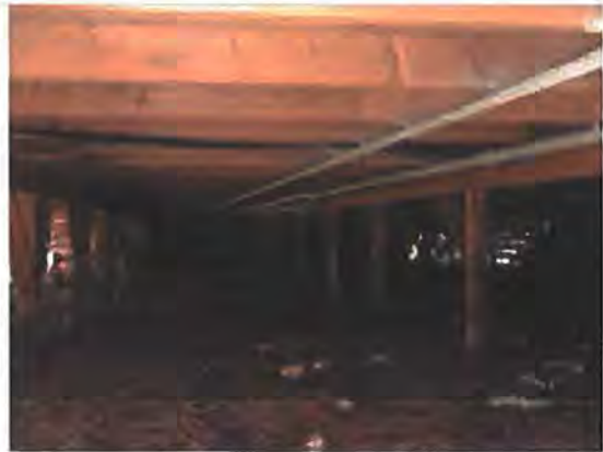
Photo 2 – Beams, girders, and sheathing from original construction
