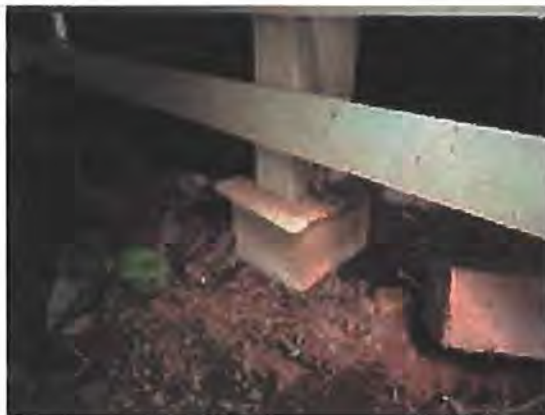
Photo 3 – Post and tofu block added during 1994 renovation
