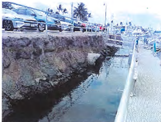
Culverts Discharging into Harbor
