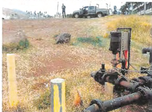
Dirt Lots with No BMPs in Place
