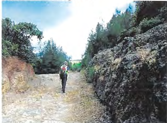
Exposed Soil Along Road
