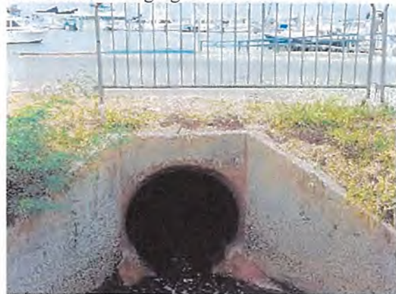
Culverts Discharging into Harbor
