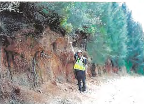
Exposed Soil Along Road
