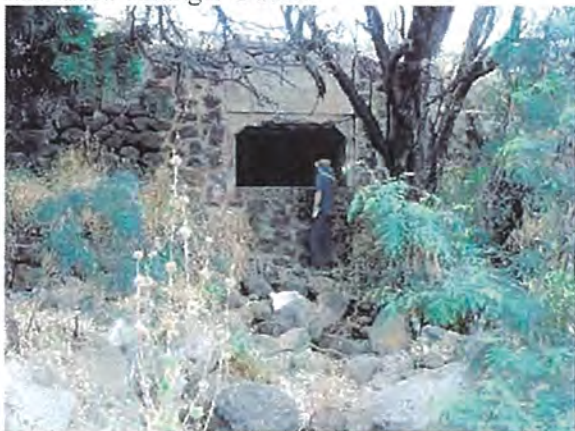
Culverts Discharging into Harbor
