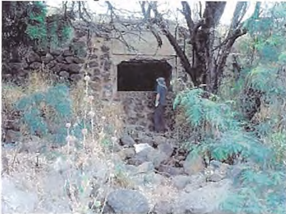
Culverts Discharging into Harbor
