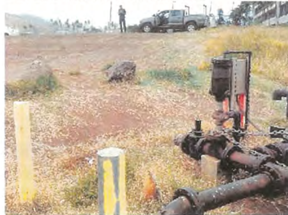
Dirt Lots with No BMPs in Place
