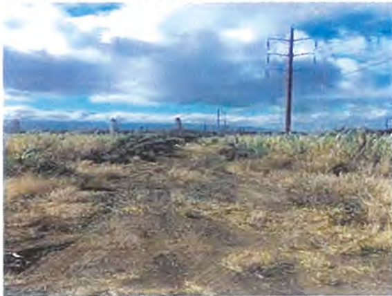
Transmission Corridor Next to Pohakea
