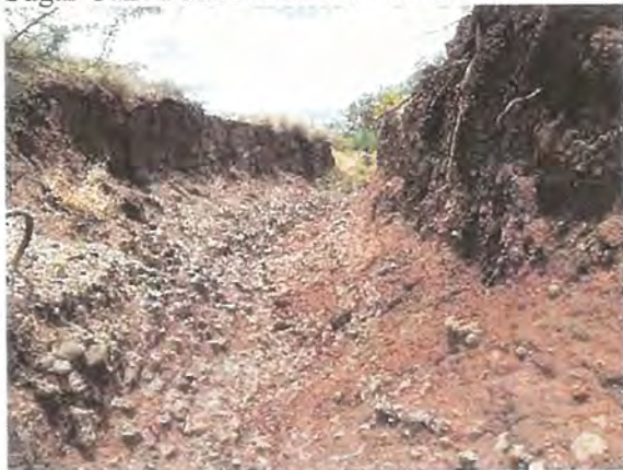
Highly Eroded Stream Channel
