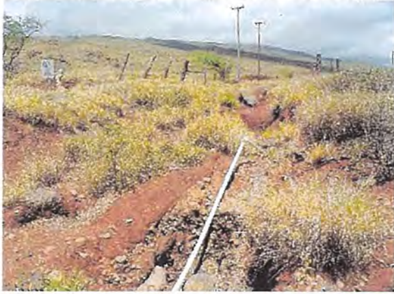
Channelization and Erosion
