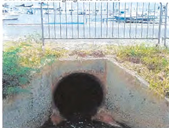
Culverts Discharging into Harbor
