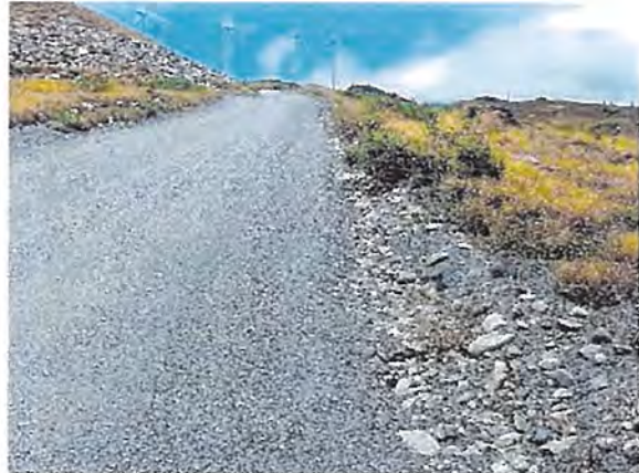
Well Maintained Road with Swale
