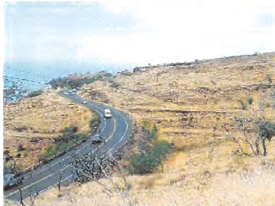
Transmission Lines along the Pali
