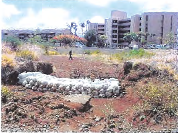
Sand Bags at Failed Control Structure
