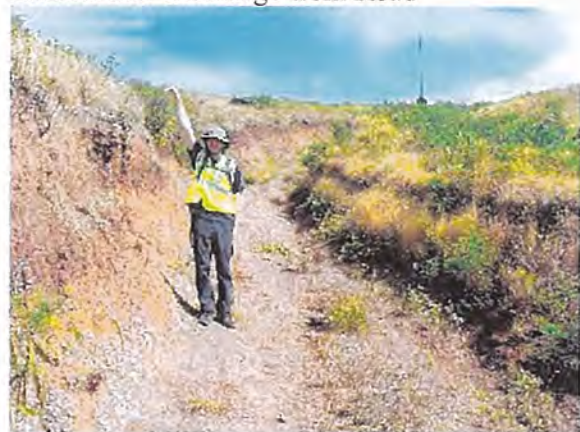
Exposed Soil Along Road
