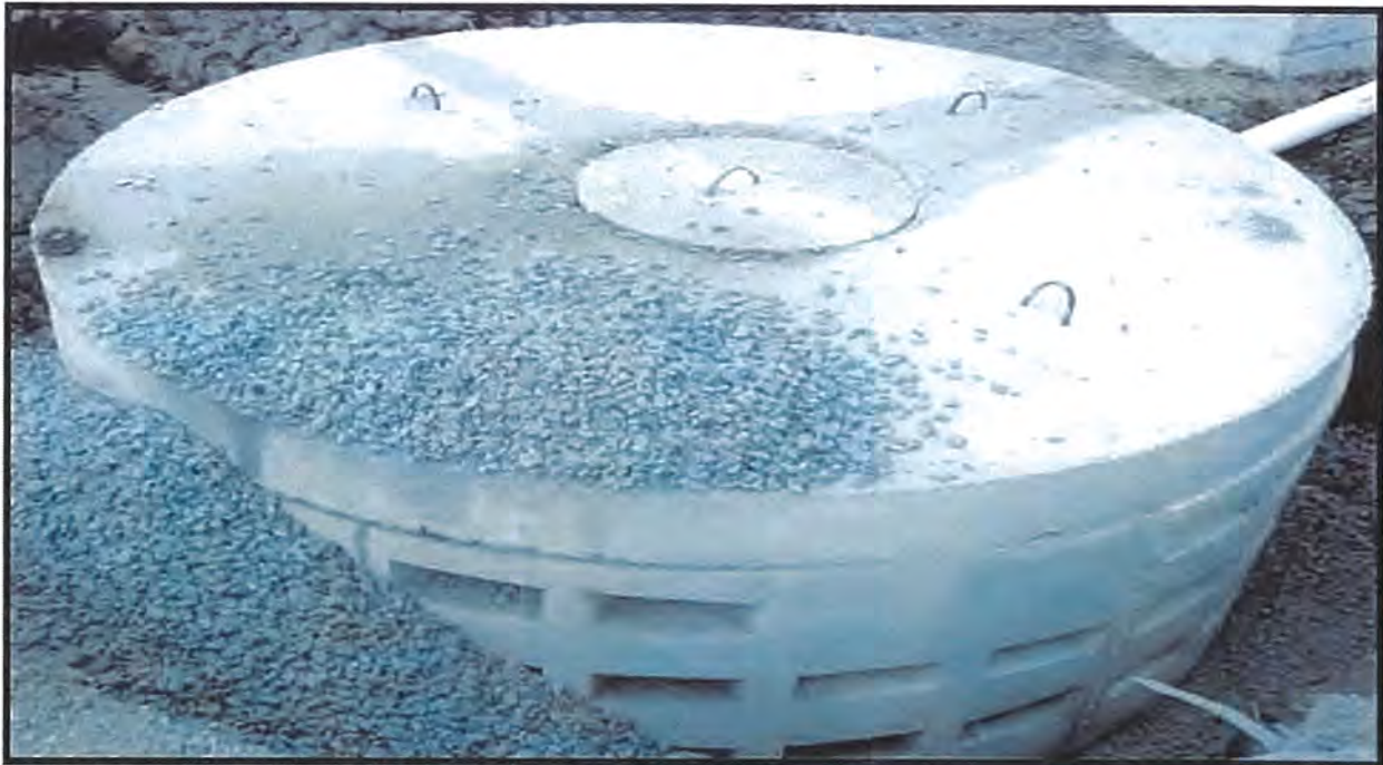
Figure 28. Stormwater Infiltration Well
