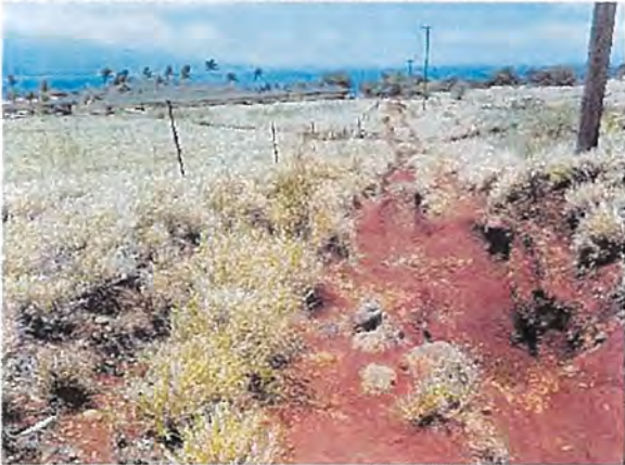
Failed Road with Channelization and Erosion
