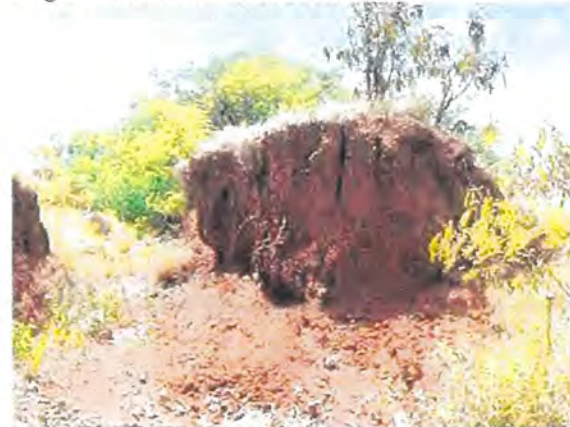
Evidence of Severe Erosion
