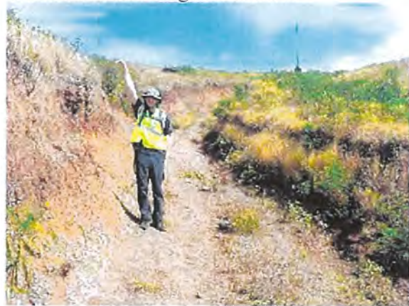
Exposed Soil Along Road
