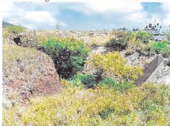
Culvert Backwall and Head Cutting
