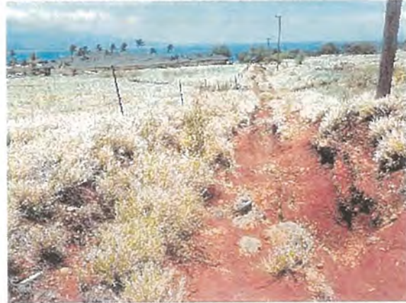
Distribution Lines and Failed Roads
