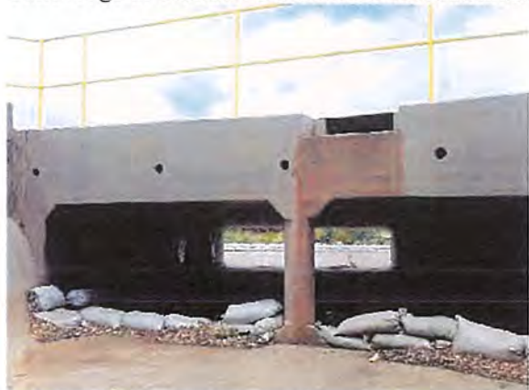
Sand Bags Under Hau'oli Street
