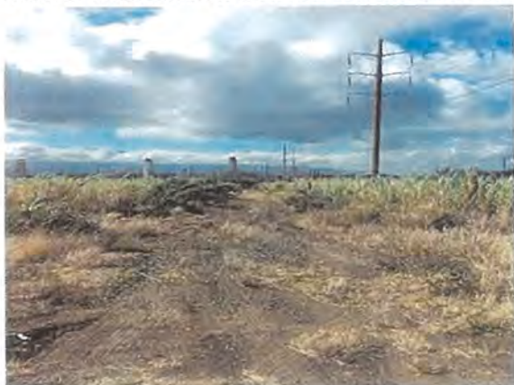
Transmission Corridor Next to Pohakea
