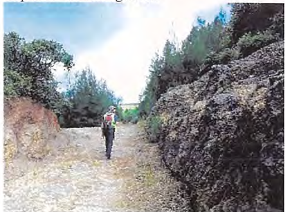
Exposed Soil Along Road
