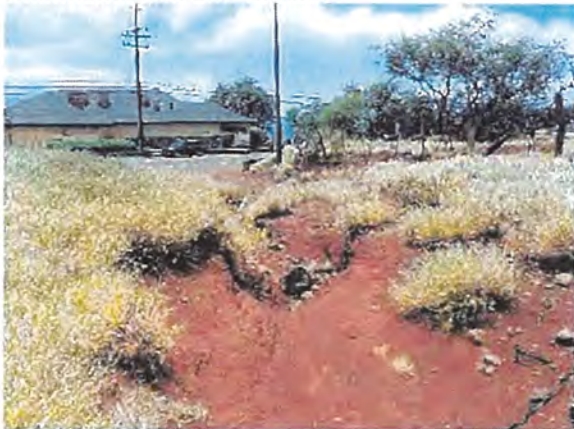
Failed Road with Channelization and Erosion
