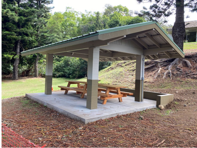
Keokea Pavilion Rebuild
