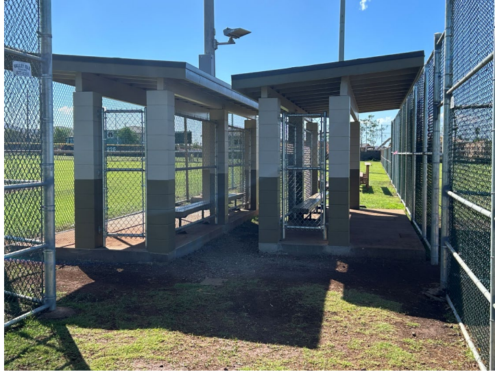
Lahaina Recreation 1 And 2 Dugout Rebuild
