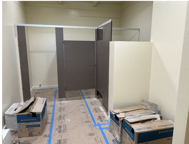
Waiehu Golf Course Women Restroom Remodel
