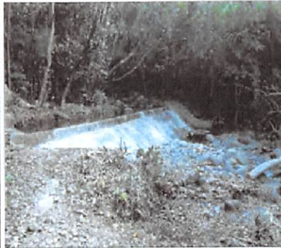
Figure 28: S. Waikapū Dam Intake Diversion (2012)
