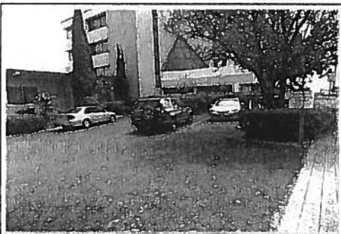
VIEW OF PARKING
