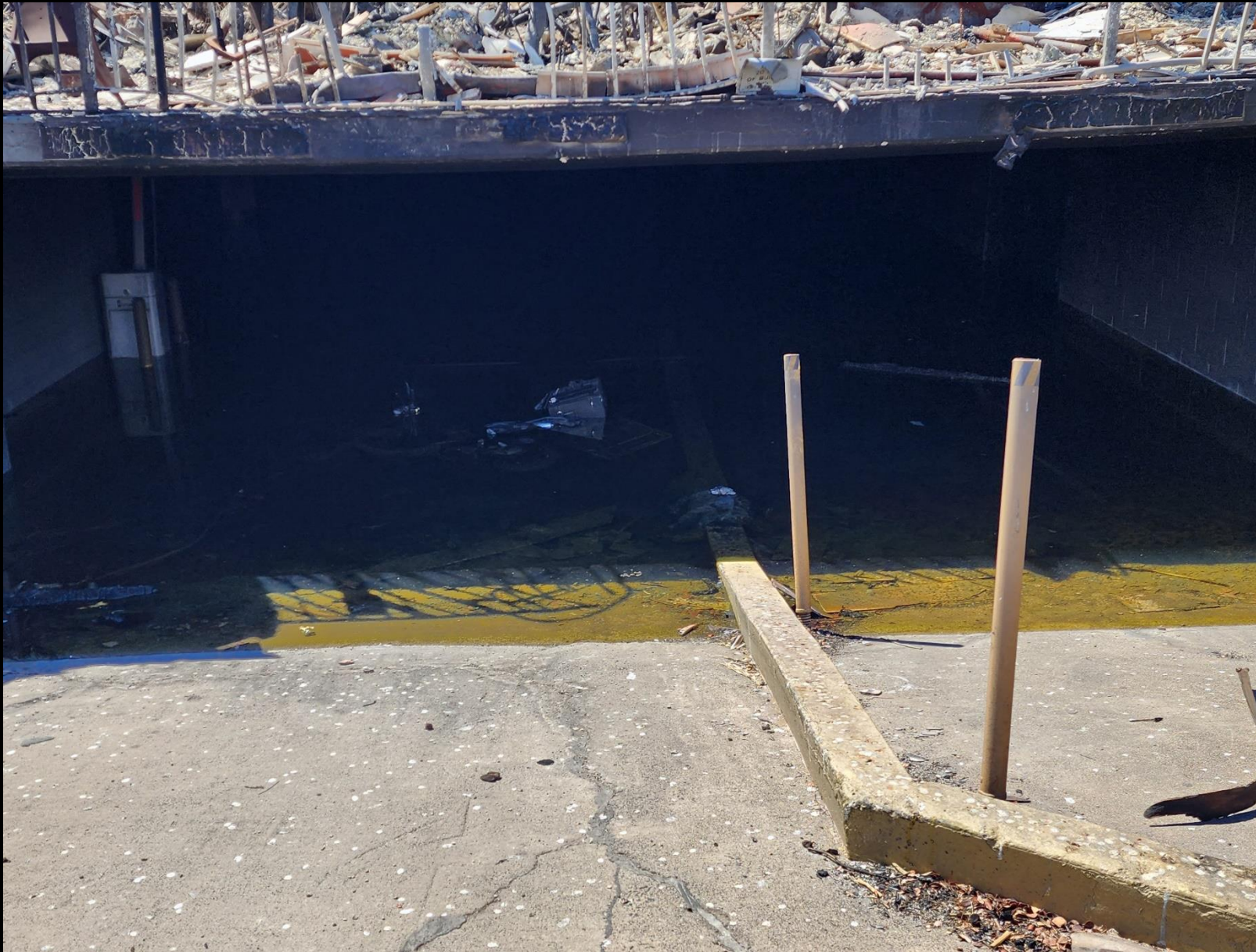
Subterranean Parking Garage 505 Front Street taken 11/1/2023
