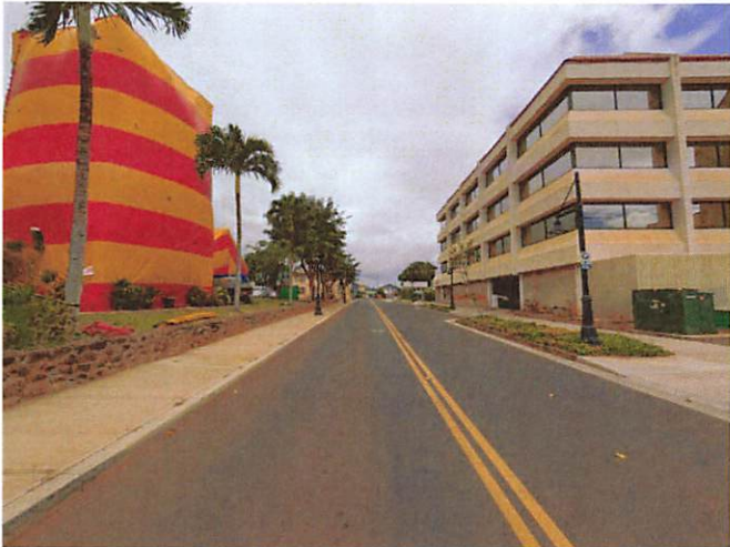
Northern View Along Church Street
