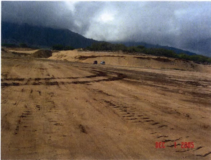
AMERON SAND EXCAVATION SITE AT MAUI LANI
