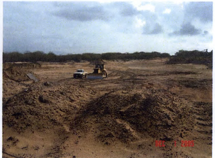
HAWAIIAN CEMENT SAND EXCAVATION SITE ON A & B's LOT 12-A
