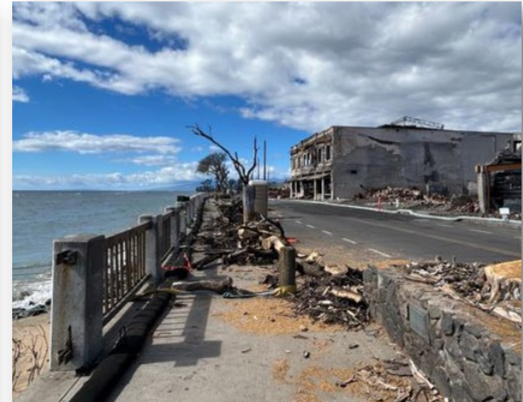
Front Street railing damaged
