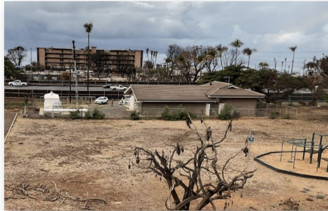
P.S. 3 – extensive wind and fire damage
