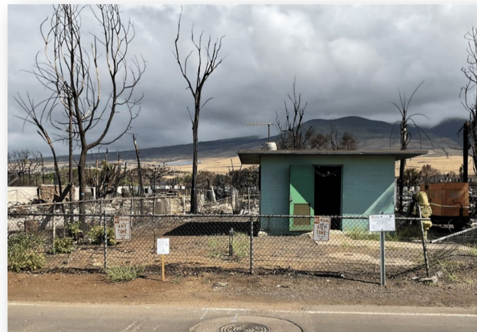
P.S. 4 – extensive wind and fire damage
