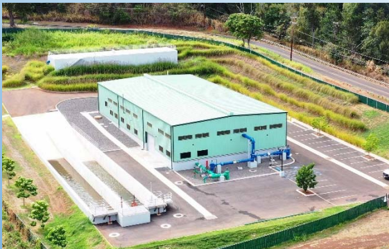
Water Treatment Facilities
