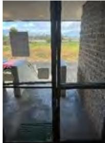
A total of 383 exterior door locations were identified in the project that could benefit from the addition of weather stripping and closure adjustments. Photos show some of the worst conditions. Note that daylight is visible around the doors. Sealing these openings will reduce the air leakage through these doors.
