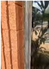
There are cracks and holes found at the window systems. These gaps allow air to find its way into the wall and window frame cavities or directly from outside to inside resulting in unwanted energy losses.
