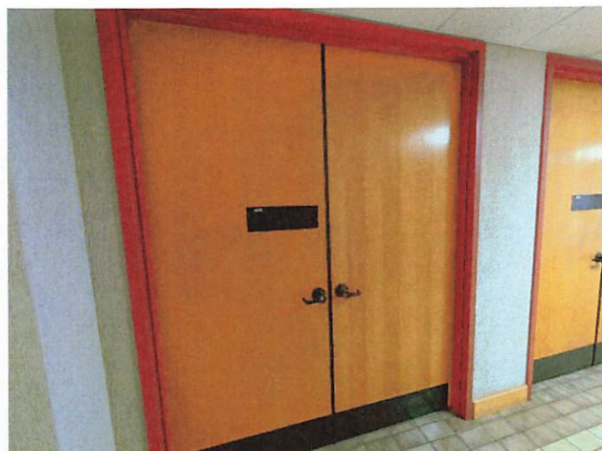
Typical Unit Entry Door
