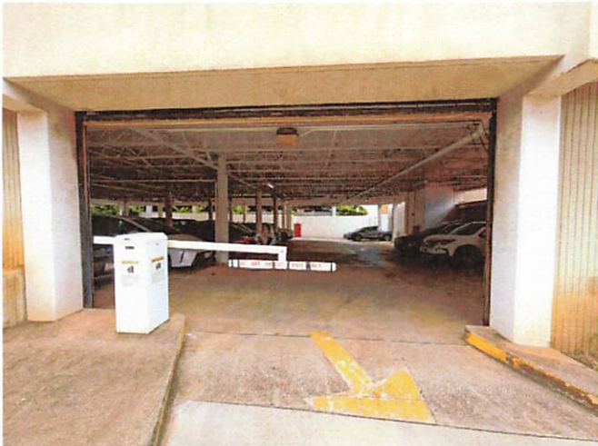
Parking Garage Egress
